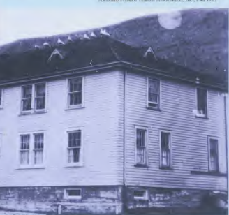
October 1943, the location of the Coast Guard Auxiliary, a hospital hospital in Unalakleet. The structure shown is the present site of the City of Unalakleet, Alaska. The Alaska Native Service Hospital, completed in 1943, is a two-story wood frame structure, measuring roughly 100 feet by 100 feet. The building stands on a small peninsula with a view of the harbor. Photo courtesy: Alaska Native Service Hospital.
