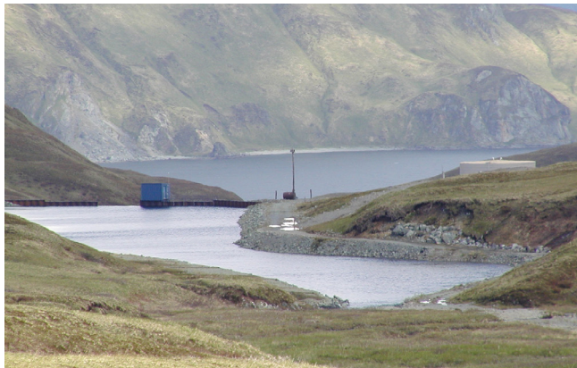
Extending the water main along Captain's Bay Road would remove a bottleneck in the water system and allow the City to use the Icy Creek Reservoir (pictured here) and Pyramid WTP to their fullest potential.
