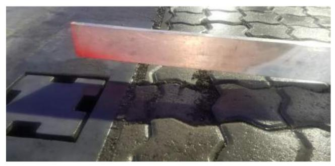
Paver blocks exceed allowable height tolerance
