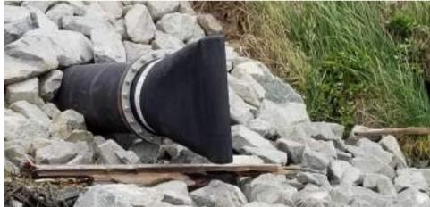
This is where the storm water drains into Margaret's Bay. The end of the pipe has a 'Tide Flex' valve to keep water from backing up into the pipe.
