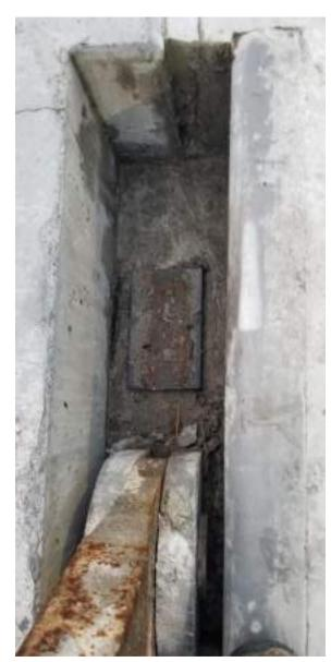
Crane Tie-Down Vault with no drain.
