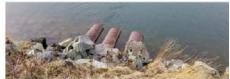
Existing Culverts are Failing
