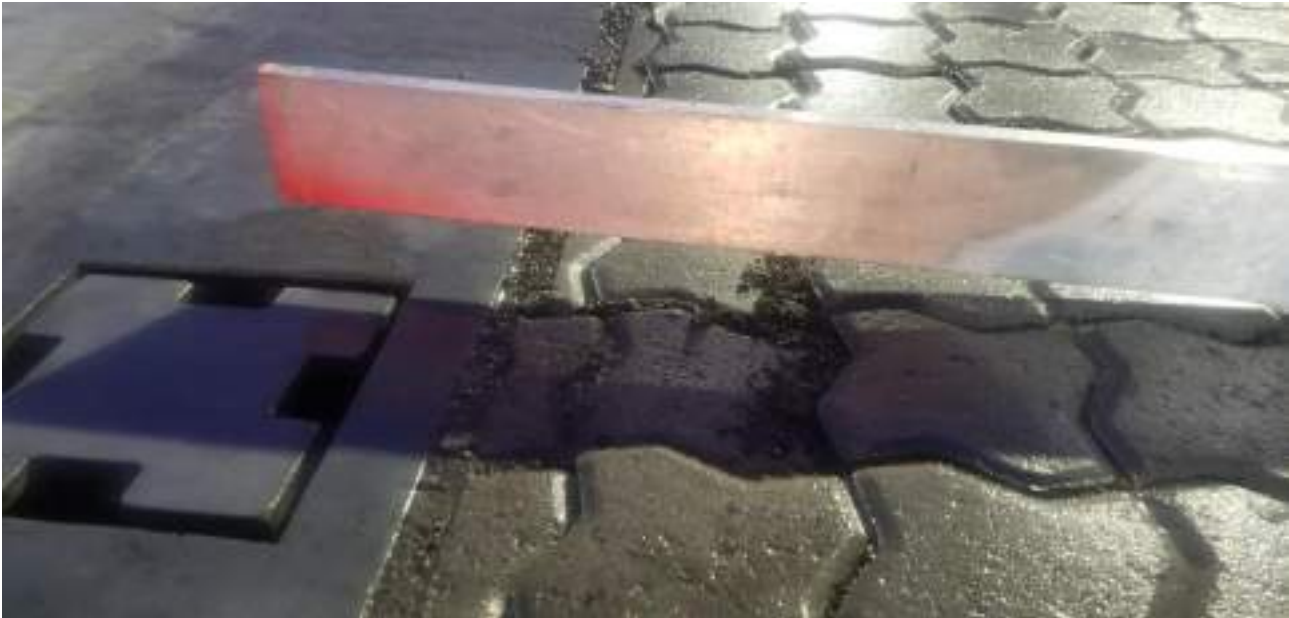
Paver blocks exceed allowable height tolerance
