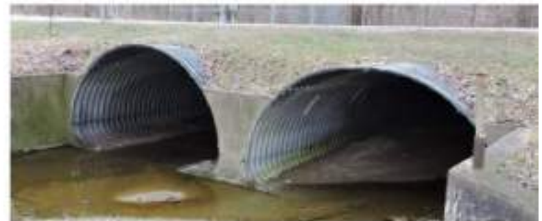
Existing Culverts are Failing
