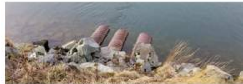
Existing Culverts are Failing
