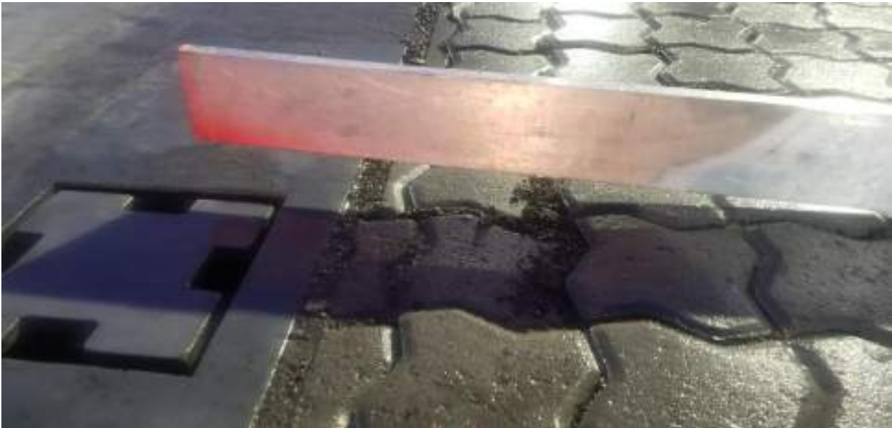
Paver blocks exceed allowable height tolerance
