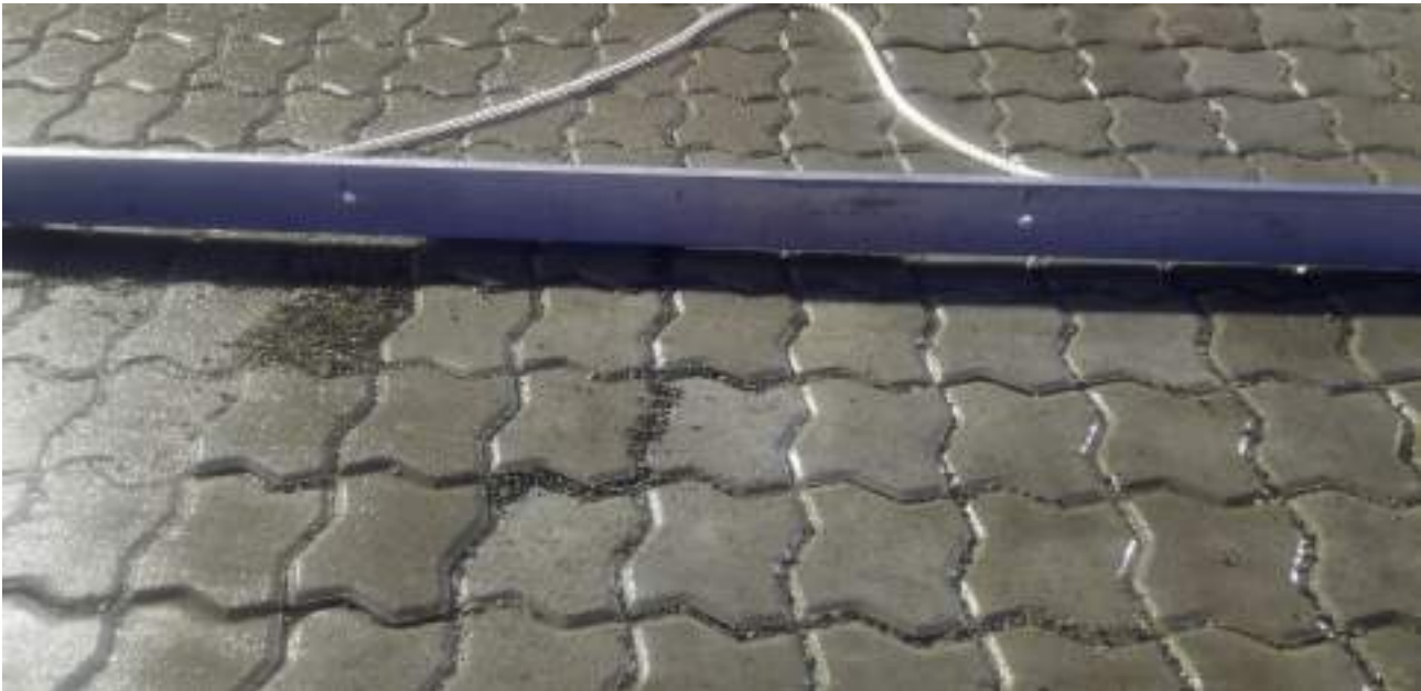
Paver blocks exceed allowable height tolerance
