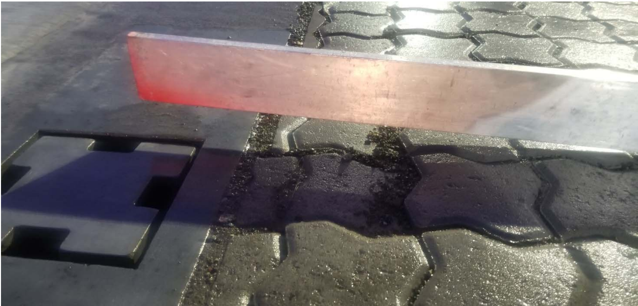
Paver blocks exceed allowable height tolerance
