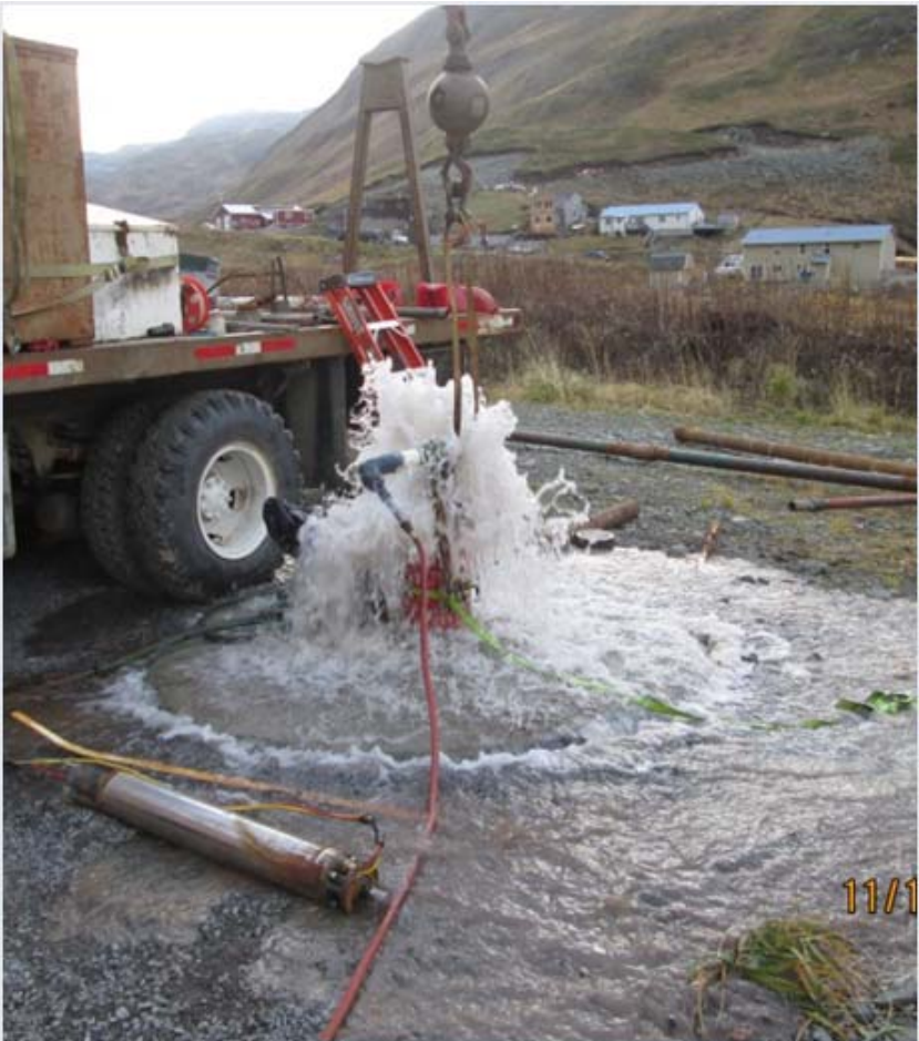
Well 2 – Replace pump & motor. Thoroughly flushed out .
