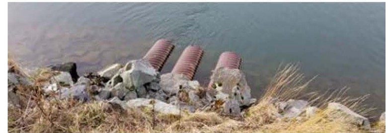
Existing Culverts are Failing
