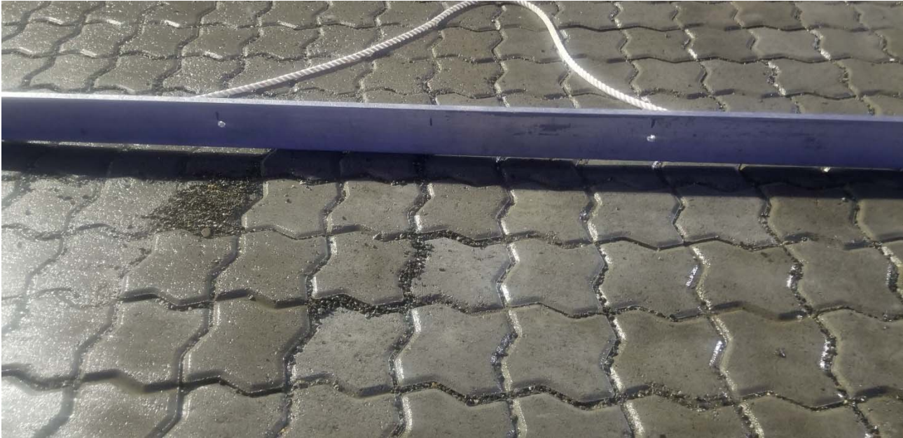
Paver blocks exceed allowable height tolerance
