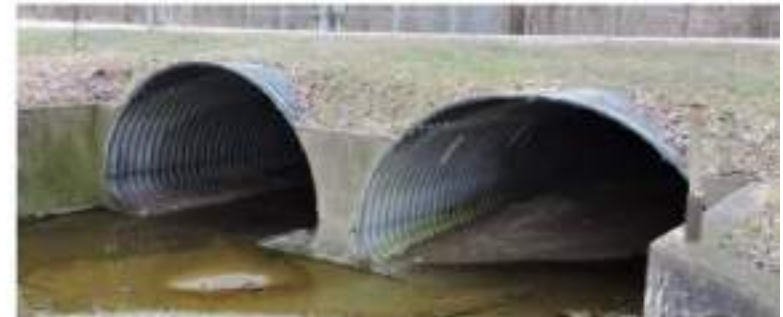
Existing Culverts are Failing
