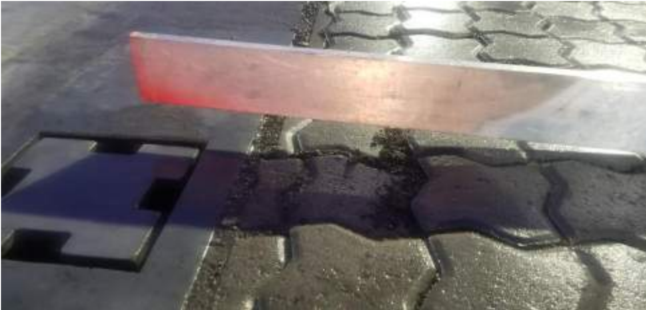
Paver blocks exceed allowable height tolerance
