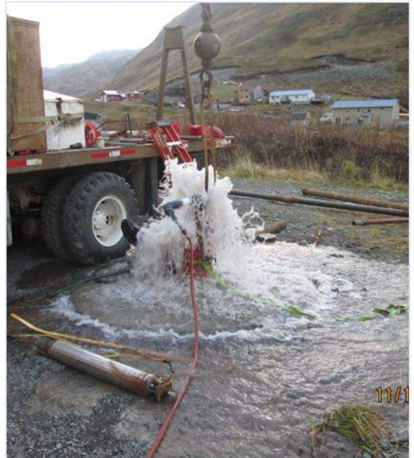
Well 2 – Replace pump & motor. Thoroughly flushed out .
