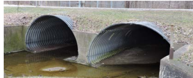
Existing Culverts are Failing
