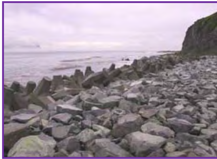
Figure 5-5 Precast Concrete Dolosse (DNR 2009)
