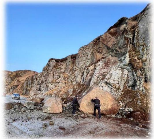
Figure 1: Three boulders totaling 36 tons fell on CBR in March 2023
