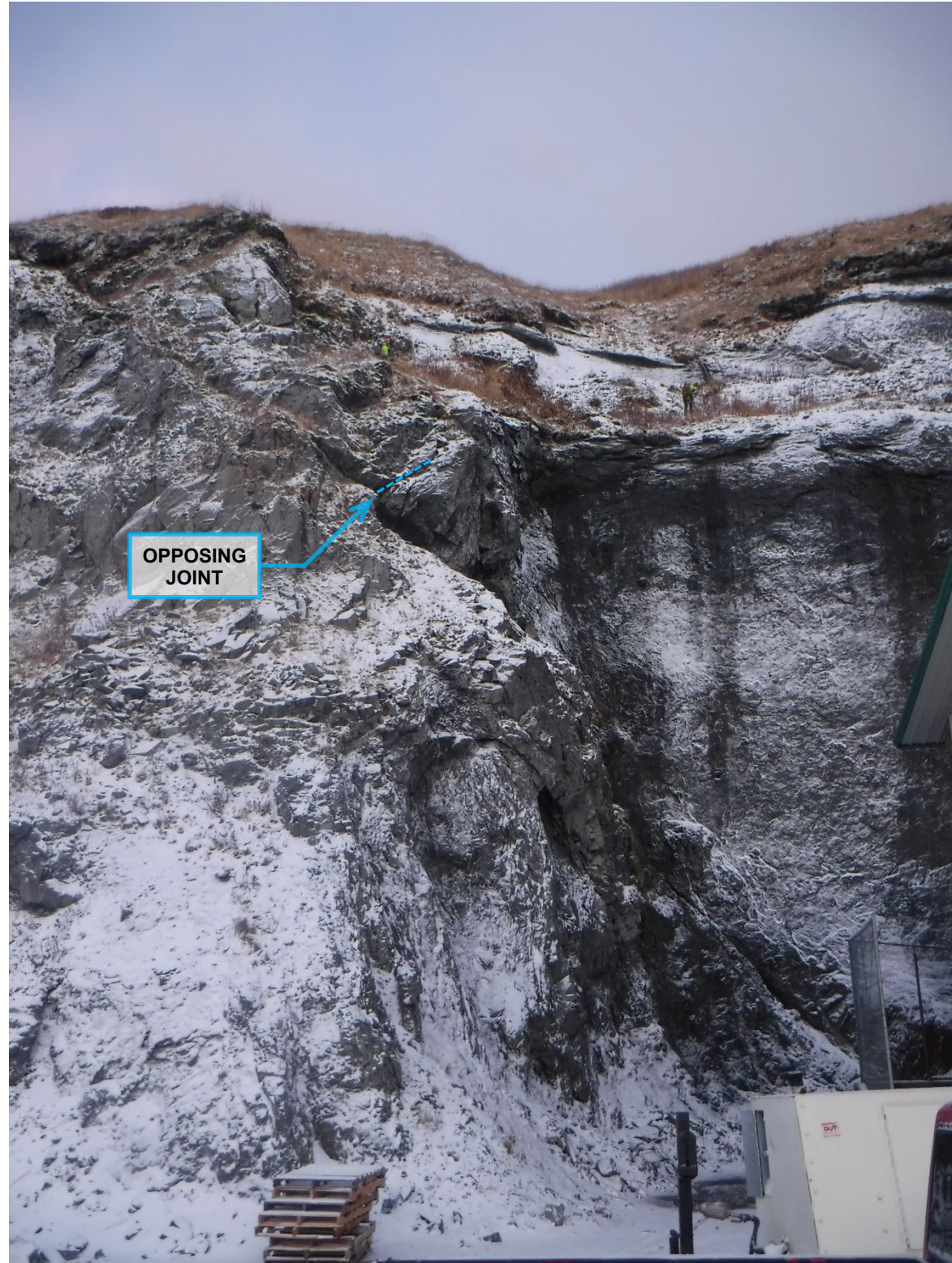
Description: Scaling Progress Photo Date: Dec 07, 2023
