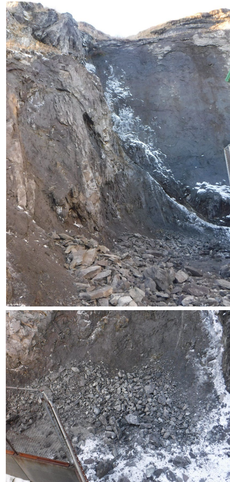
Description: Scaling Progress and Accumulations of Rocks Scaled Off the Face (WU 1a, CSL) After Day 1. Photo Date: Dec 05, 2023
