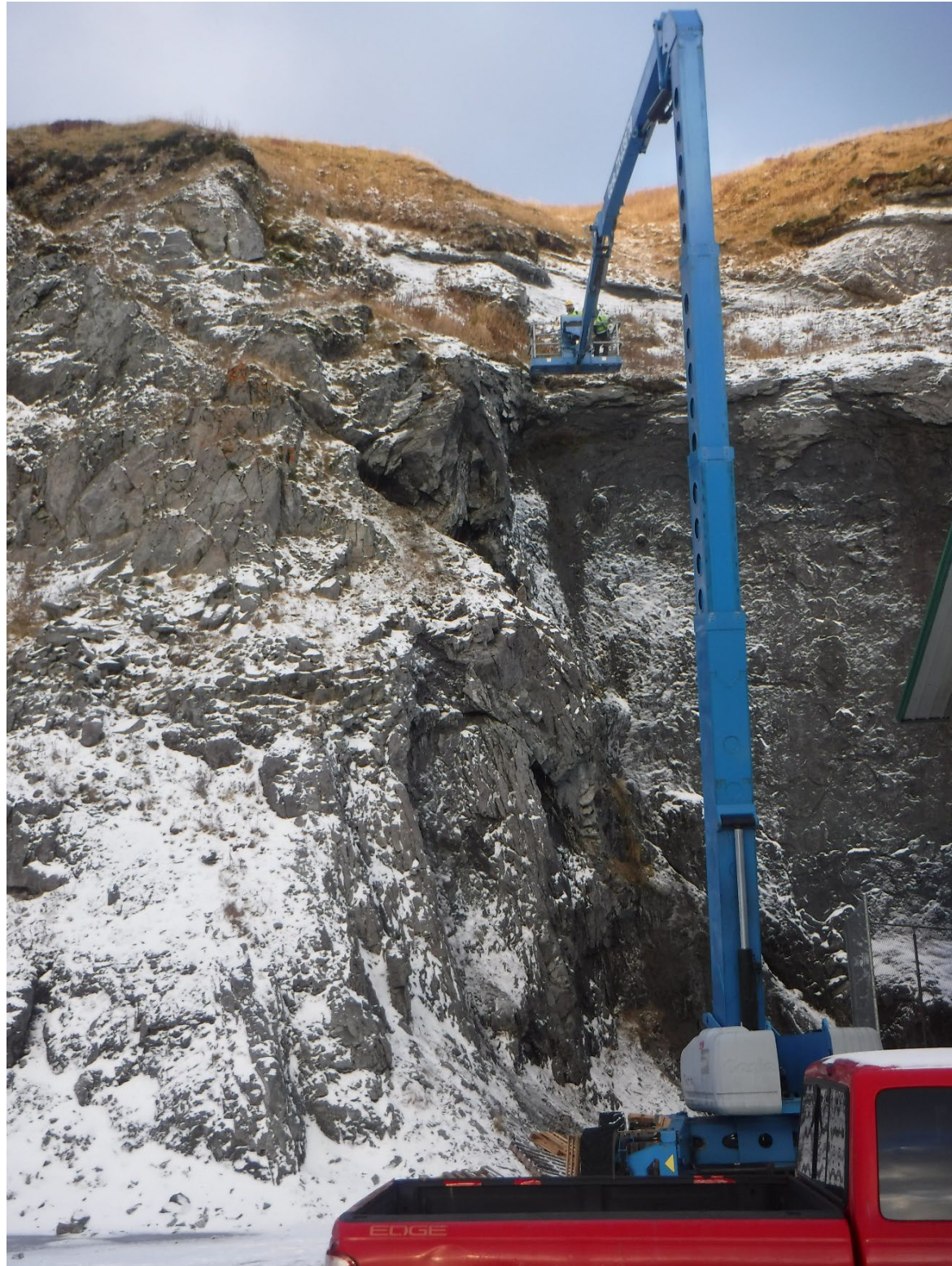
Description: Day 1 Scaling Operations at WU 1a Via Manlift Photo Date: Dec 05, 2023
