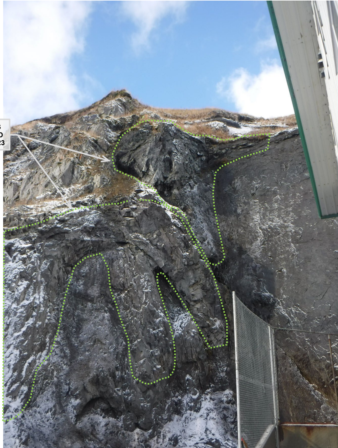
Description: Condition and Outline of Completed Scaling Photo Date: Dec 07, 2023
