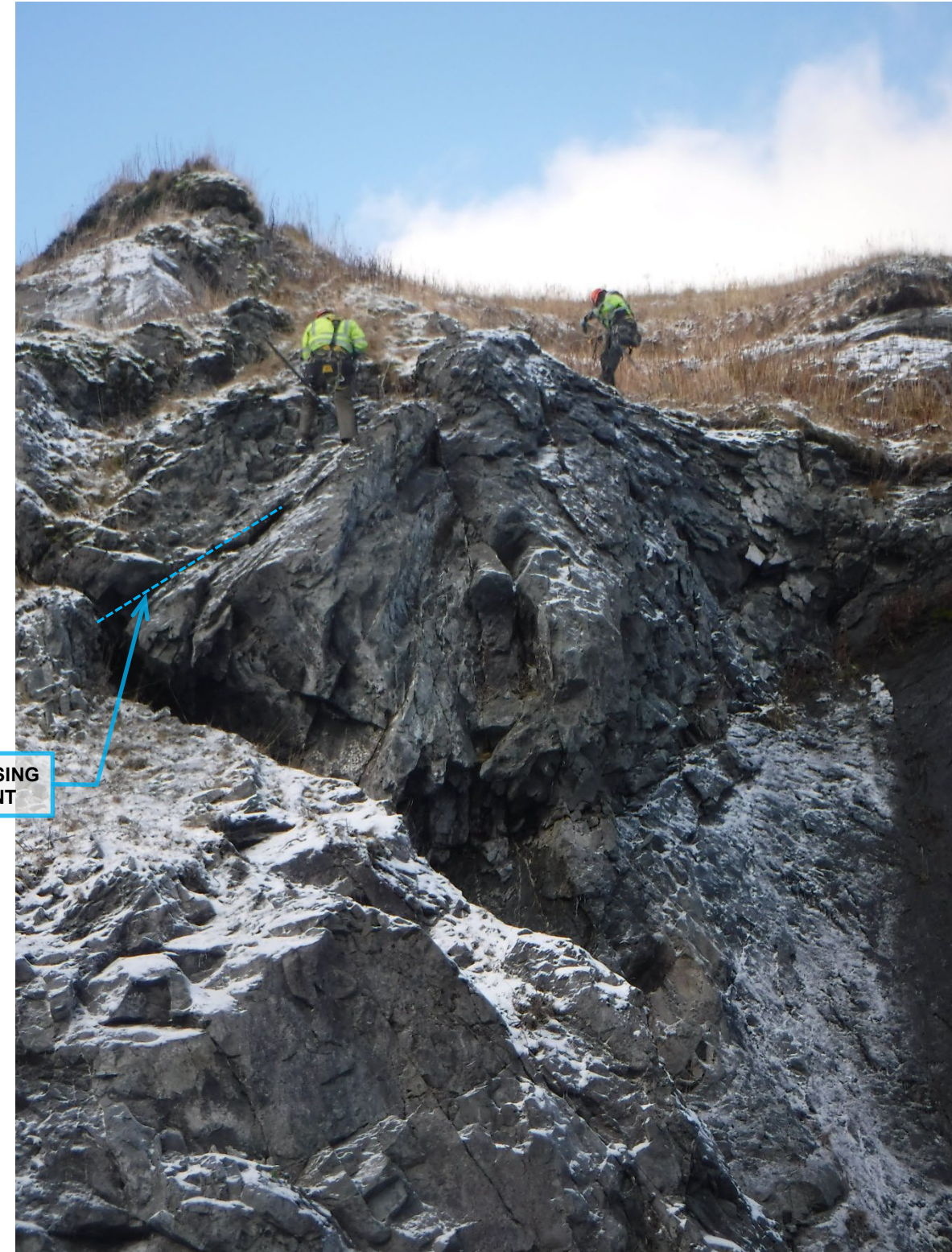
Description: Scaling Progress Upper Wedge Photo Date: Dec 07, 2023
