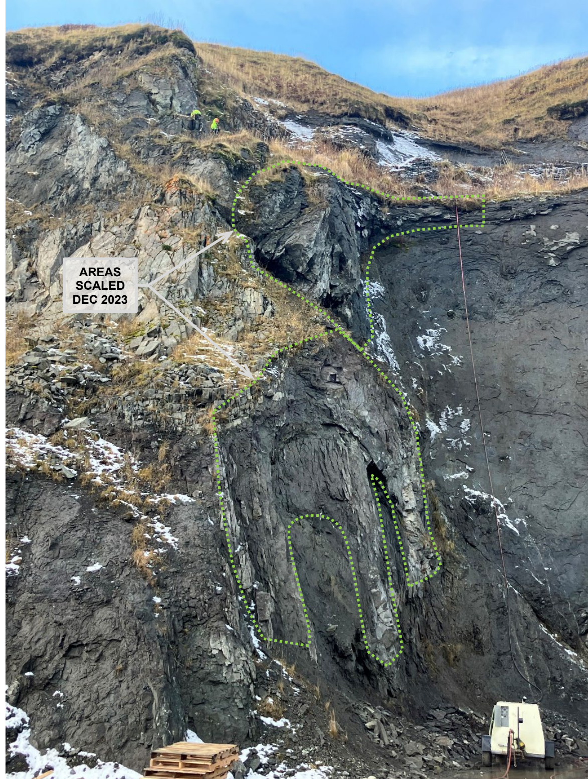
Description: Condition and Outline of Completed Scaling Photo Date: Dec 06, 2023
