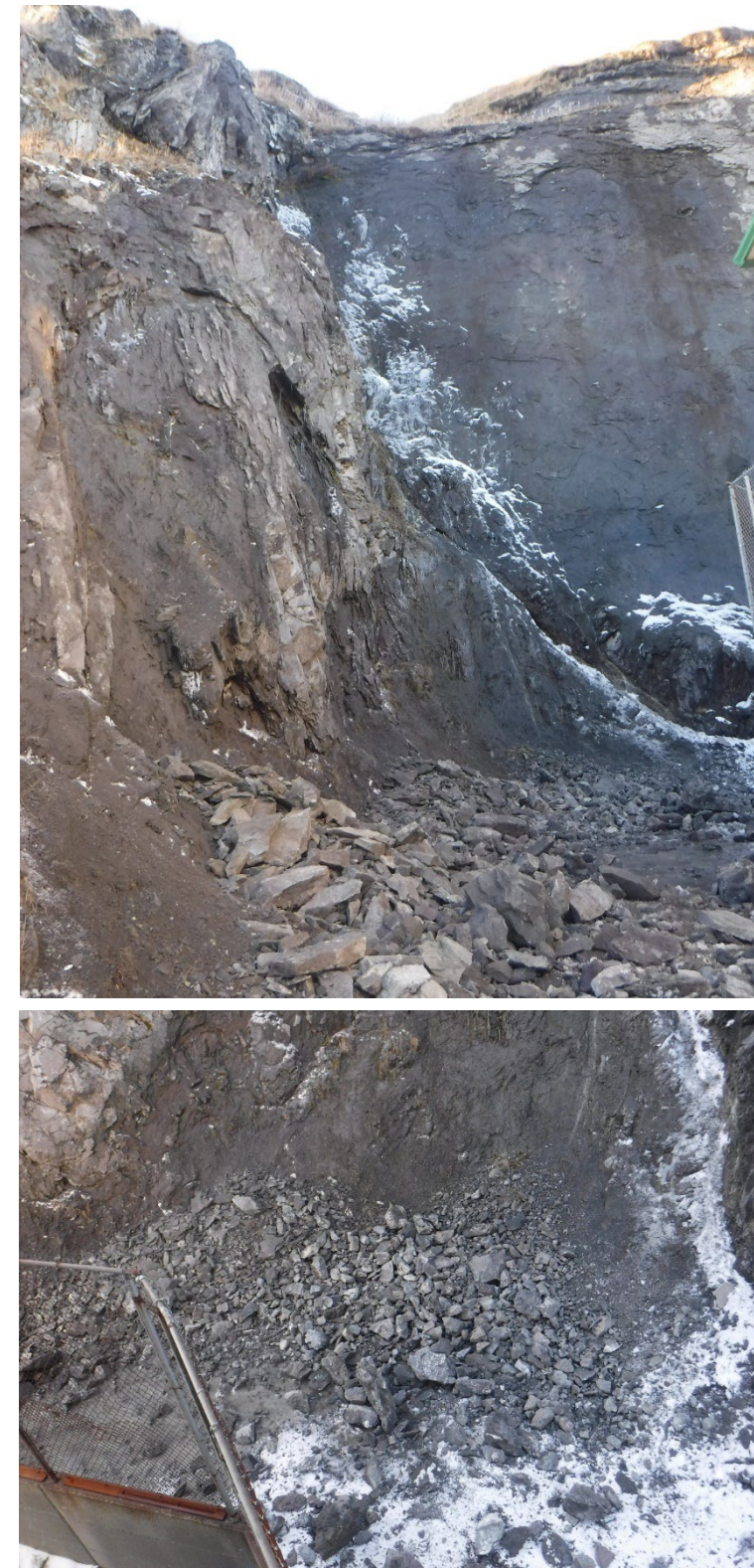
Description: Scaling Progress and Accumulations of Rocks Scaled Off the Face (WU 1a, CSL) After Day 1. Photo Date: Dec 05, 2023
