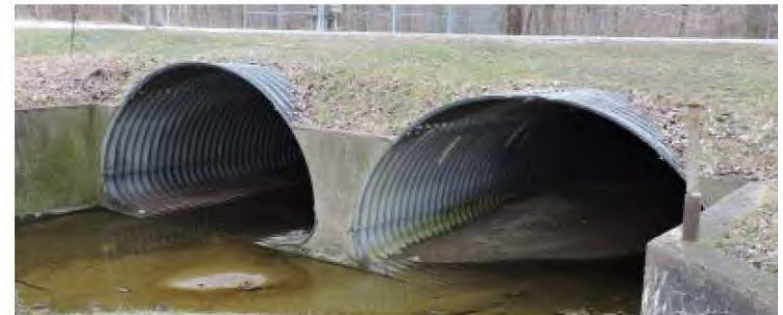
Existing Culverts are Failing
