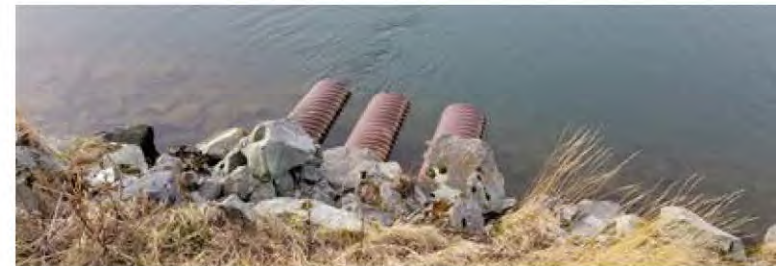
Existing Culverts are Failing
