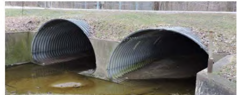
Existing Culverts are Failing
