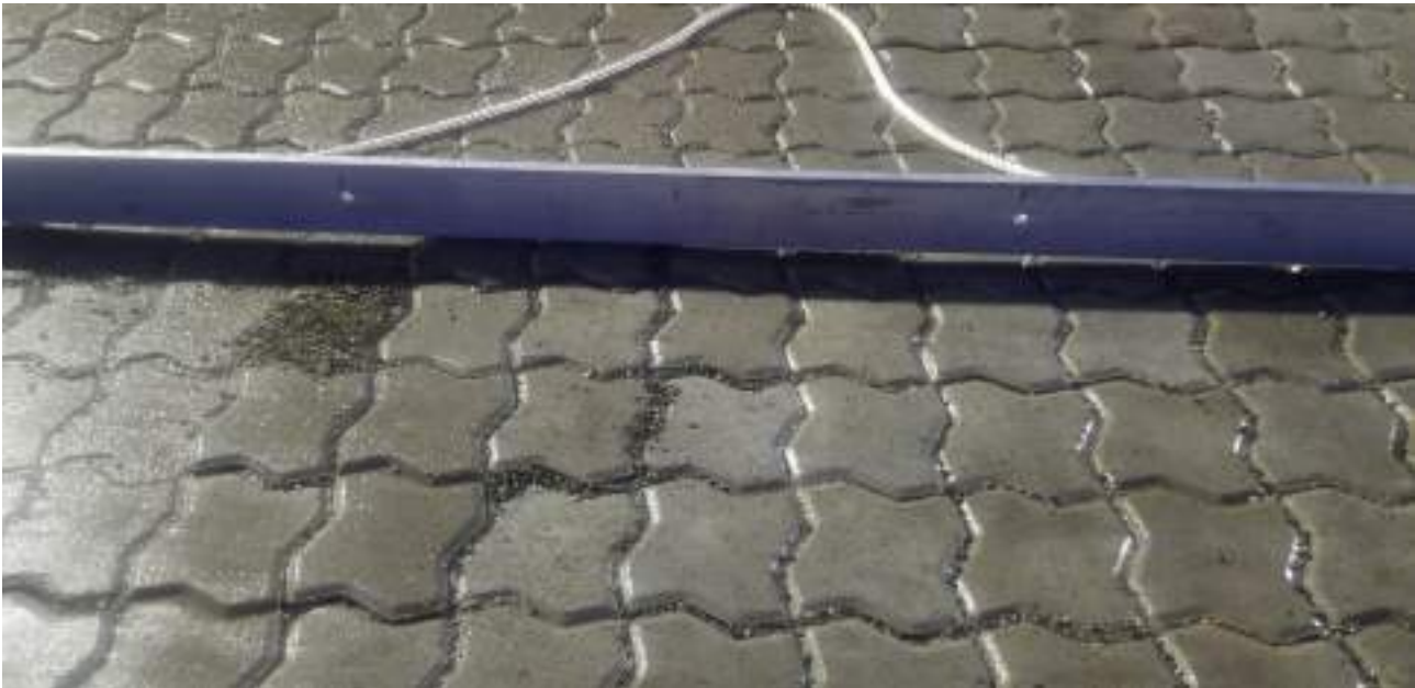
Paver blocks exceed allowable height tolerance
