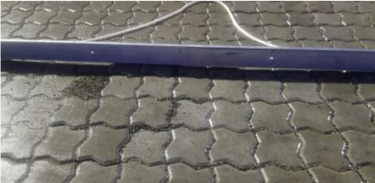
Paver blocks exceed allowable height tolerance
