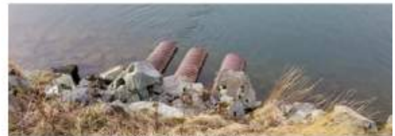
Existing Culverts are Failing
