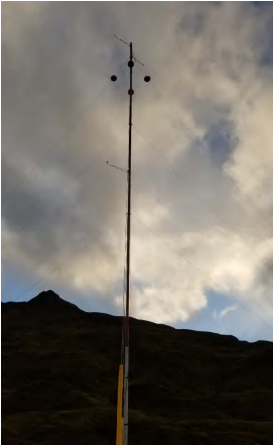
ICR 34 m, northeast side (view to southwest)
