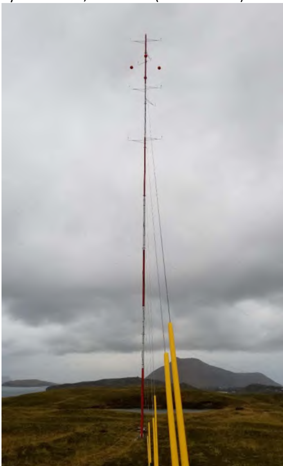
Pyramid 60 m, south side (view to north)
