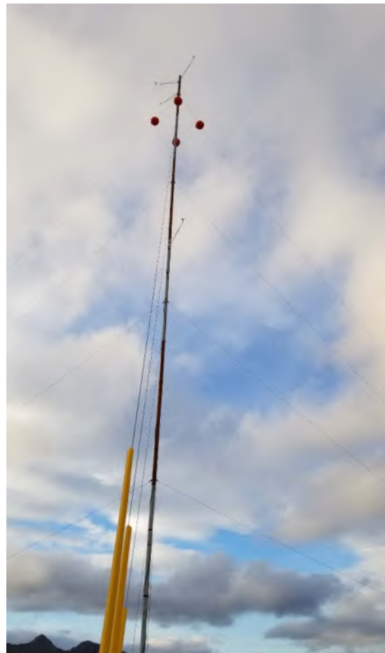
ICR 34 m, southeast side (view to northwest)
