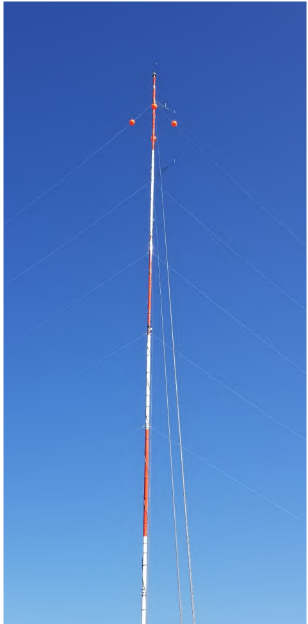
Hog island 60 m, west side (view to east)
