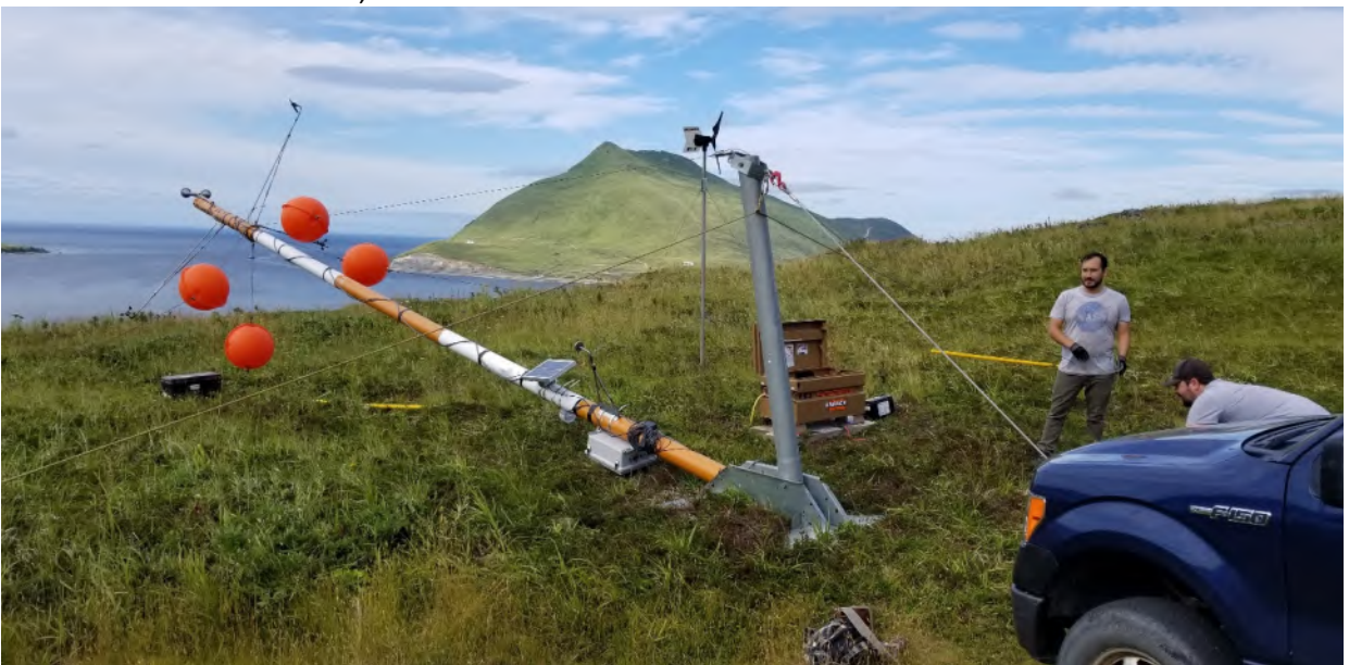
Bunker Hill 10 m met tower during installation
