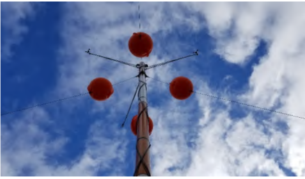
Bunker Hill 10 m, uptower, north face
