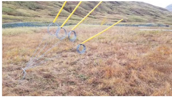
ICR 34 m, southeast anchors
