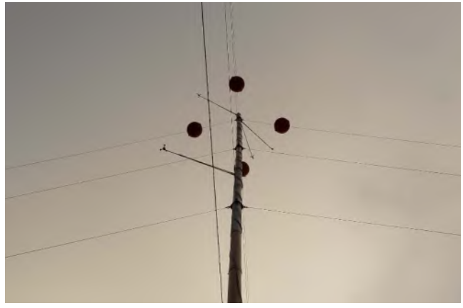
ICR 34 m, uptower, northeast face
