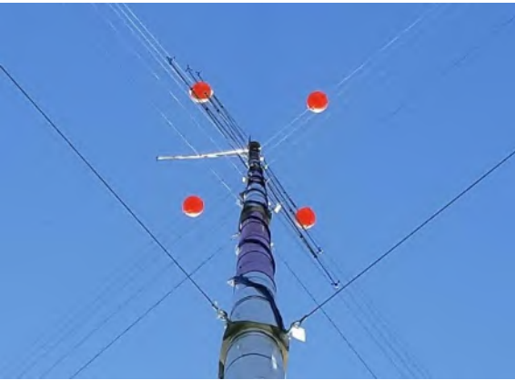
Hog Island 60 m, uptower, northeast face
