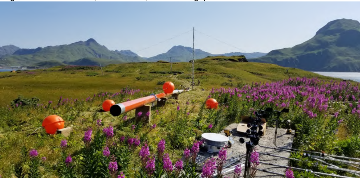
Hog Island tower during assembly, view south
