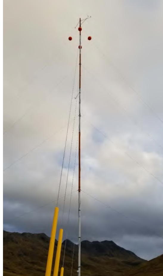
ICR 34 m, northwest side (view to southeast)
