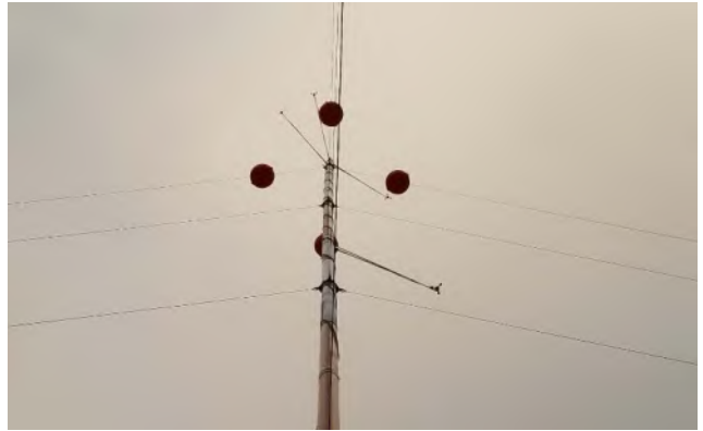
ICR 34 m, uptower, southwest face
