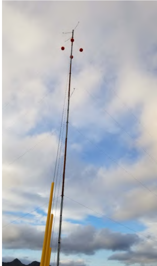
ICR 34 m, southeast side (view to northwest)
