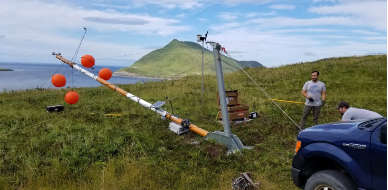
Bunker Hill 10 m met tower during installation
