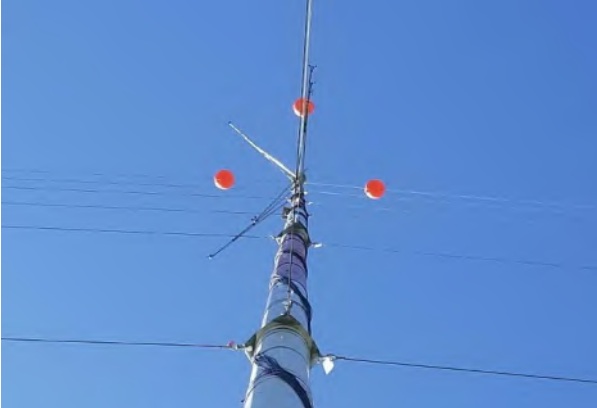
Hog Island 60 m, uptower, east face
