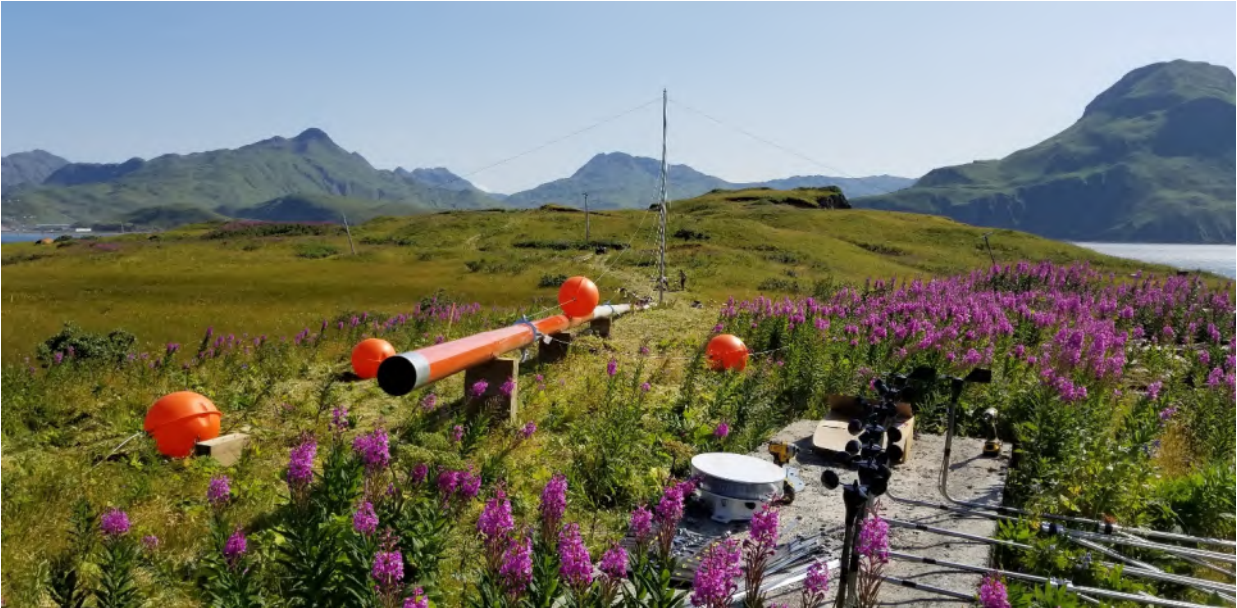
Hog Island tower during assembly, view south
