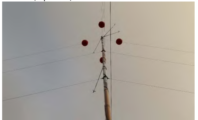
ICR 34 m, uptower, northwest face
