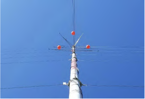
Hog Island 60 m, uptower, south face
