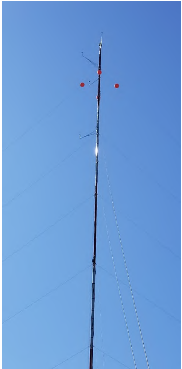
Hog Island 60 m, east side (view to west)
