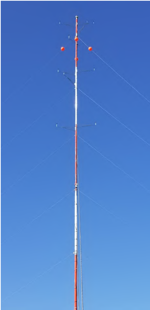
Hog Island 60 m, south side (view to north)
