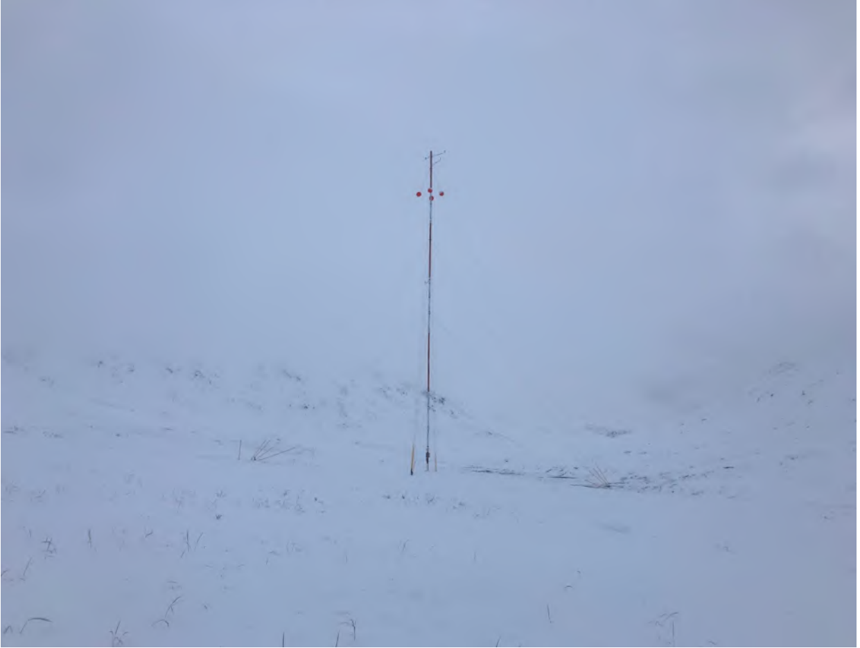
ICR 34 m met tower winter view, view to northwest (K. Arduser photo)
