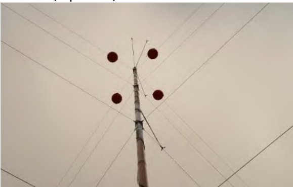
ICR 34 m, uptower, west face
