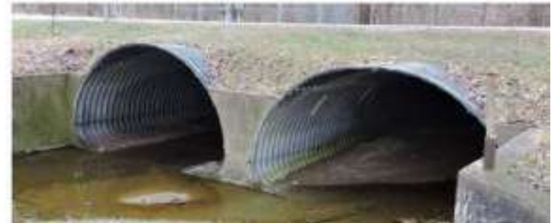
Existing Culverts are Failing
