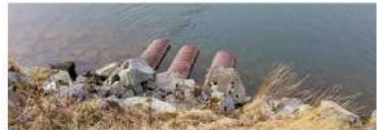
Existing Culverts are Failing
