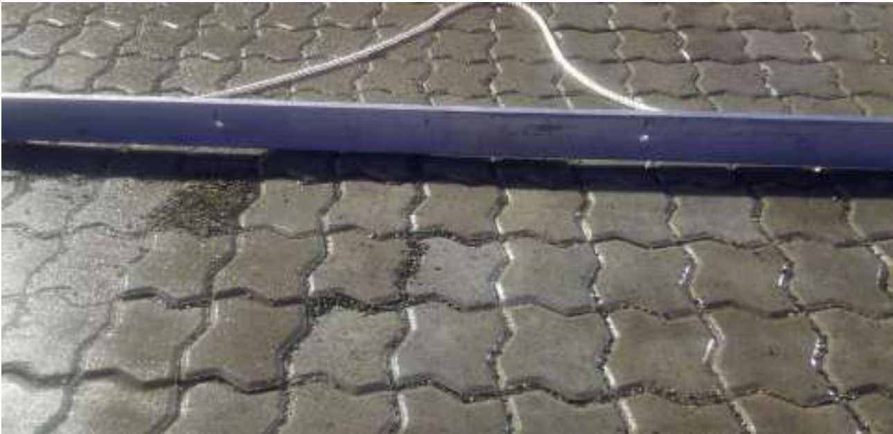
Paver blocks exceed allowable height tolerance
