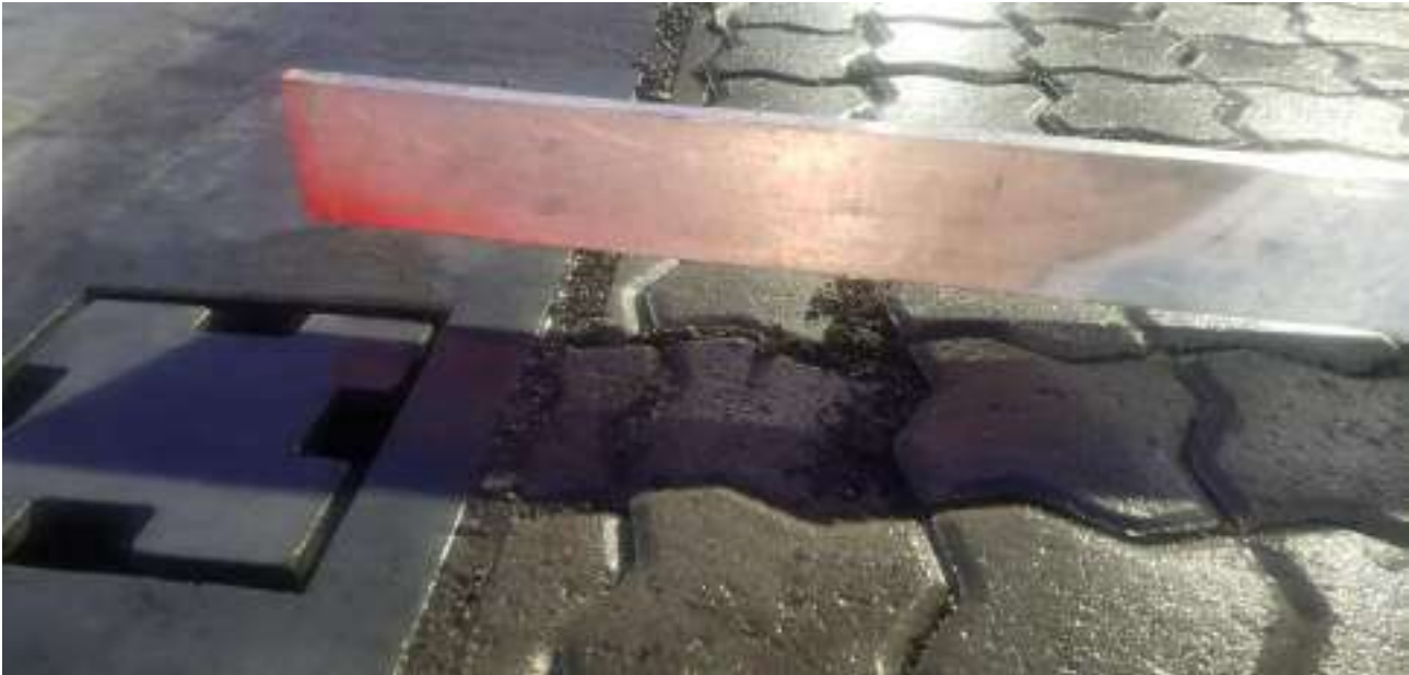
Paver blocks exceed allowable height tolerance
