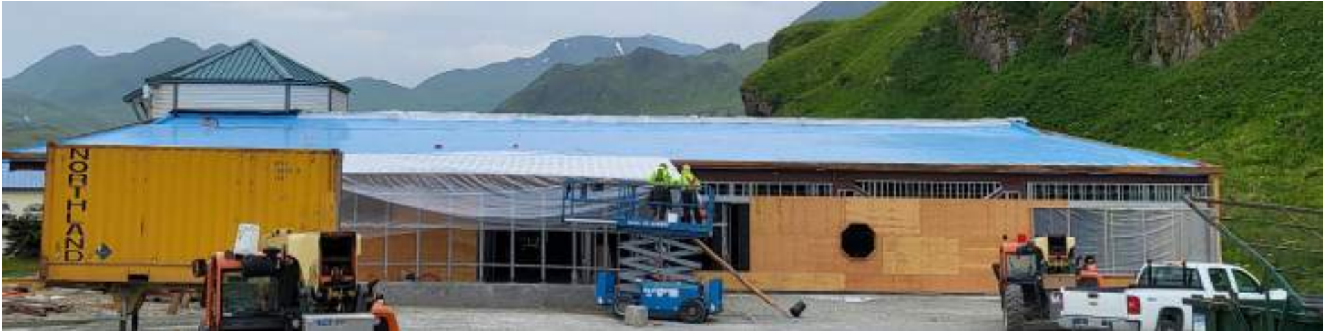
Exterior Overview on 7-20-22
