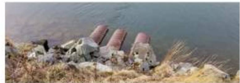
Existing Culverts are Failing
