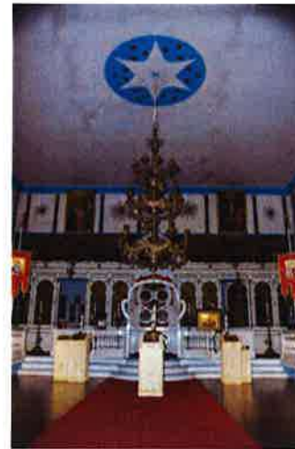
Holy Ascension Cathedral ceiling with sprinkler heads. Photo: Dave Gregory
