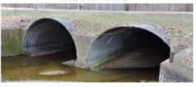
Proposed culverts improve fish habitat, can be visually inspected, and are large enough to accommodate tidal fluctuations and heavy rainfall.
