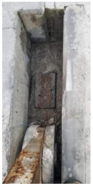
Crane Tie-Down Vault with no drain.
