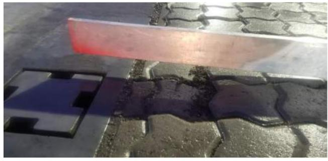
Paver blocks exceed allowable height tolerance
