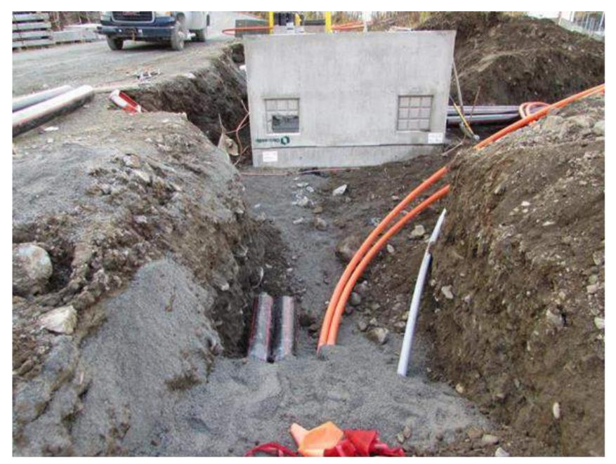
Fiber optic cable is typically laid in 2" orange conduit.
