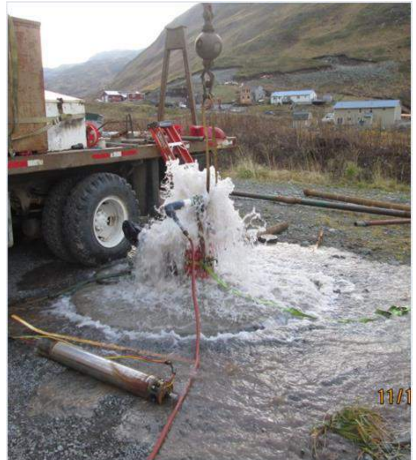
Well 2 – Replace pump & motor. Thoroughly flushed out .
