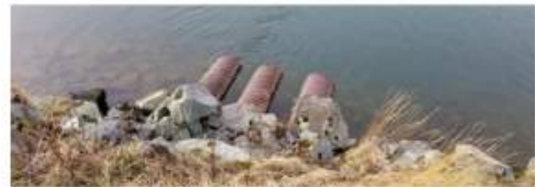
Existing Culverts are Failing
