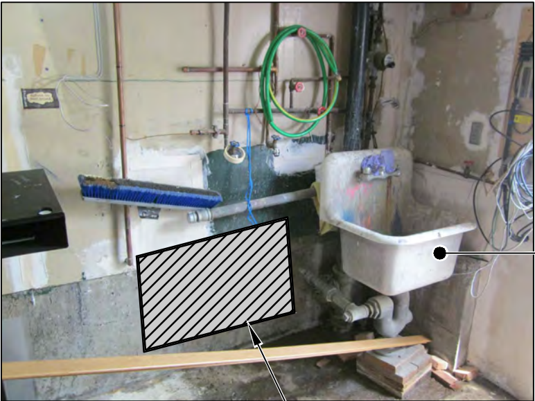
4 PHOTO 5.01 SCALE: NOT TO SCALE REMOVE AND REINSTALL SINK AS REQUIRED FOR ACCESS INSTALL METER AND RPBA IN THIS GENERAL AREA. AREA ABOVE AND TO THE LEFT OF THIS AREA MAY BE USED AS WELL.
