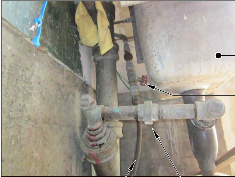
3 PHOTO 5.01 SCALE: NOT TO SCALE SINK SHUT-OFF VALVE SOFT COPPER TO UTILITY ROUTE RPBA DRAIN BEHIND SINK AND THROUGH EXTERIOR WALL
