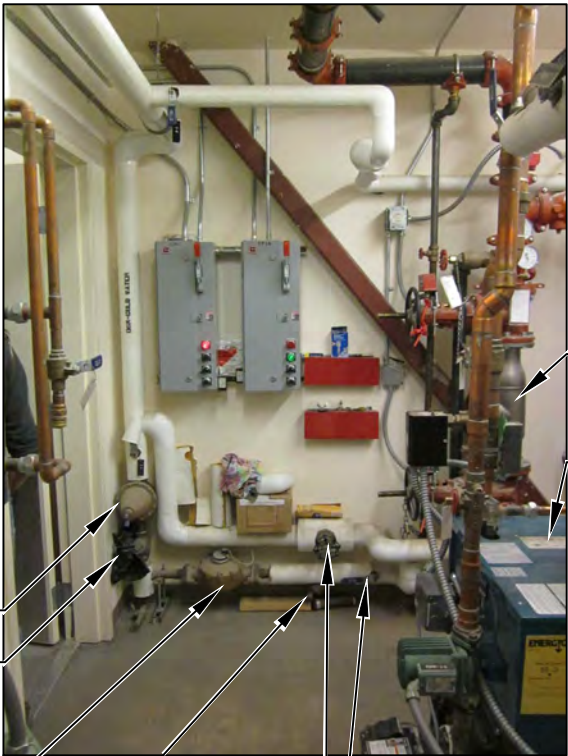
METER — STRAINER — METER BYPASS SHUT-OFF VALVE — SHUT-OFF VALVE
