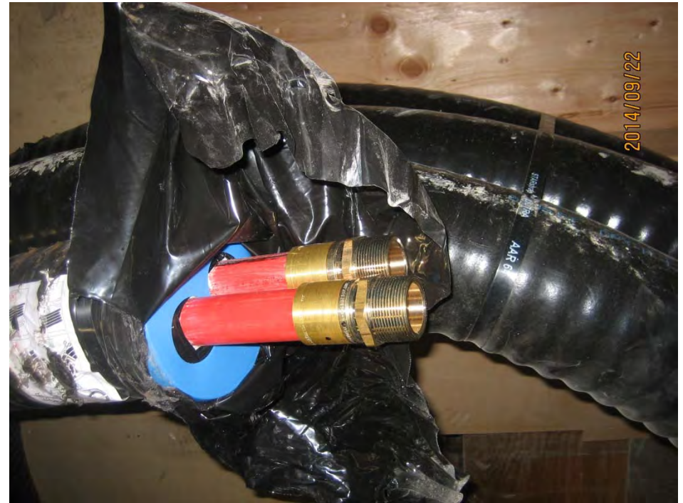
Pipe ends at junction box at time of installation in 2014.
