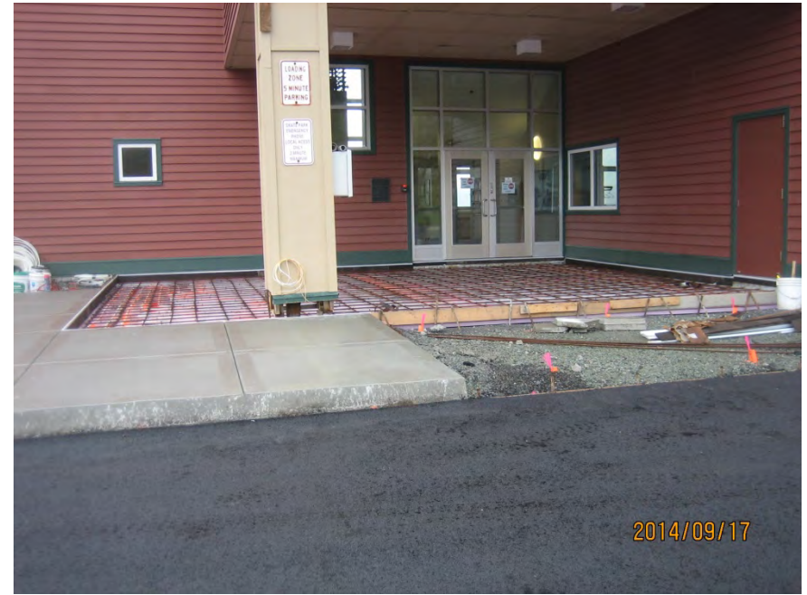
Installation of insulation and tubing for heated slab on 9-17-14.
