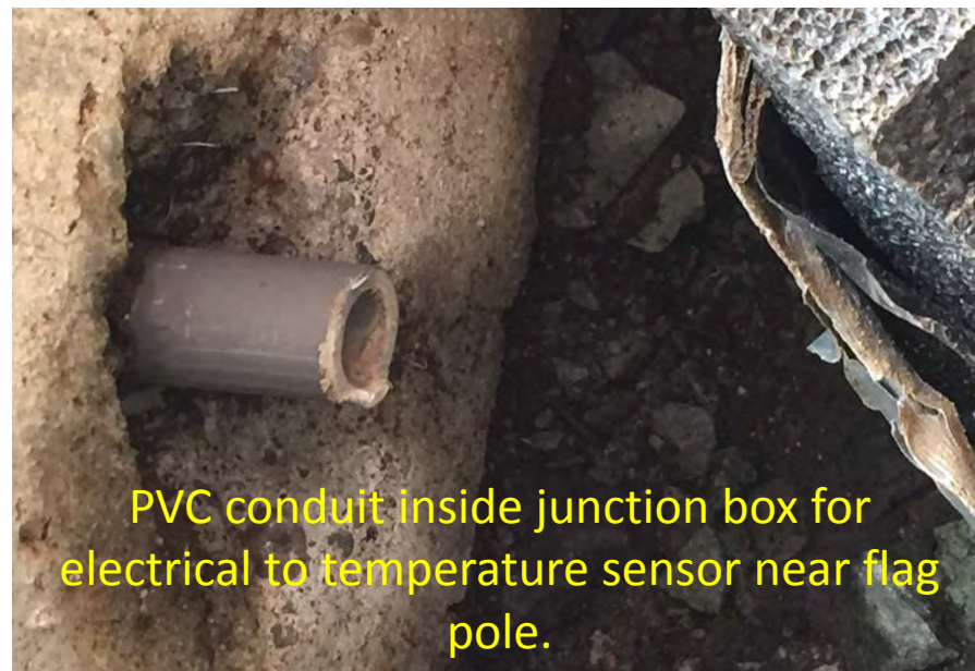
Pipe ends in junction box on 4-20-16.
