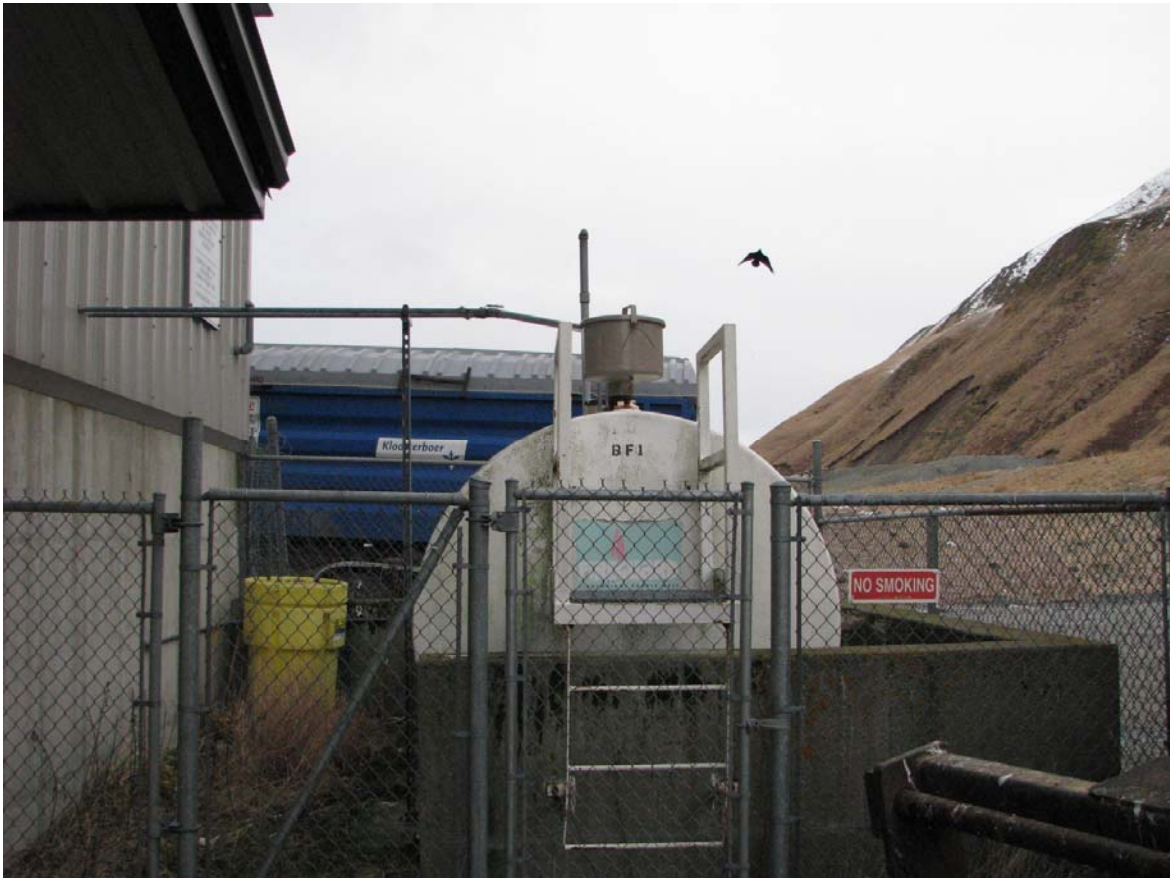
Fuel Oil Tank and Piping
