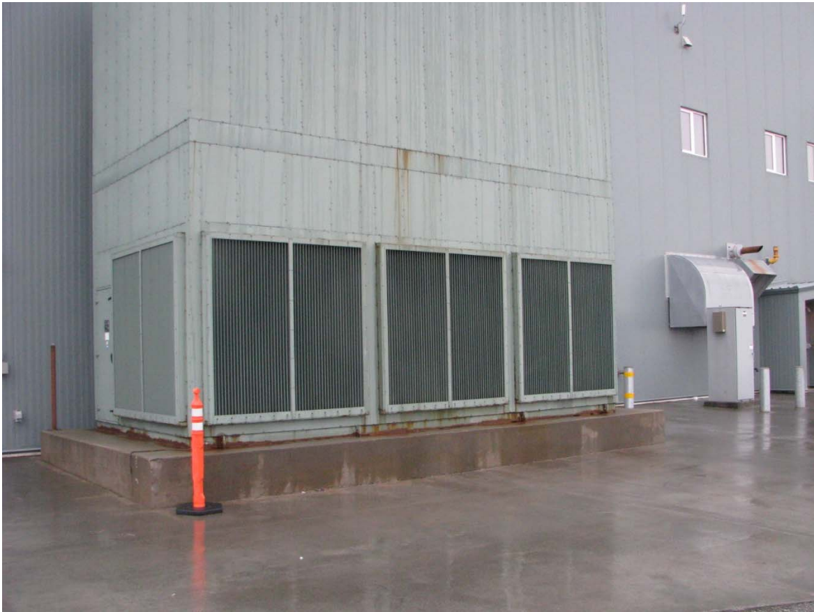
New Powerhouse – Air Handling Unit 1
