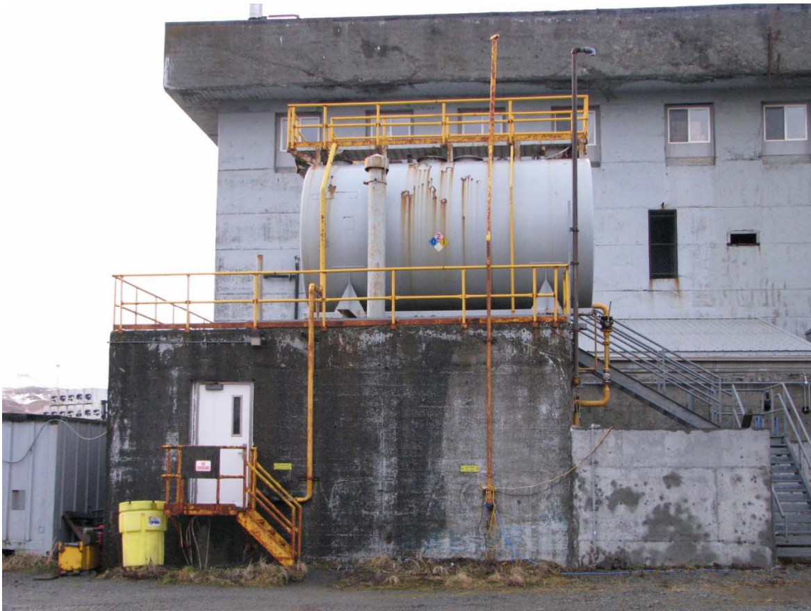
Old Powerhouse – Fuel Oil Tank, Piping, Platform Rails, Stairs, Service Platform, Misc. Steel
