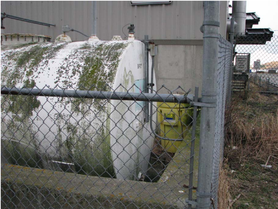
Fuel Oil Tank and Piping
