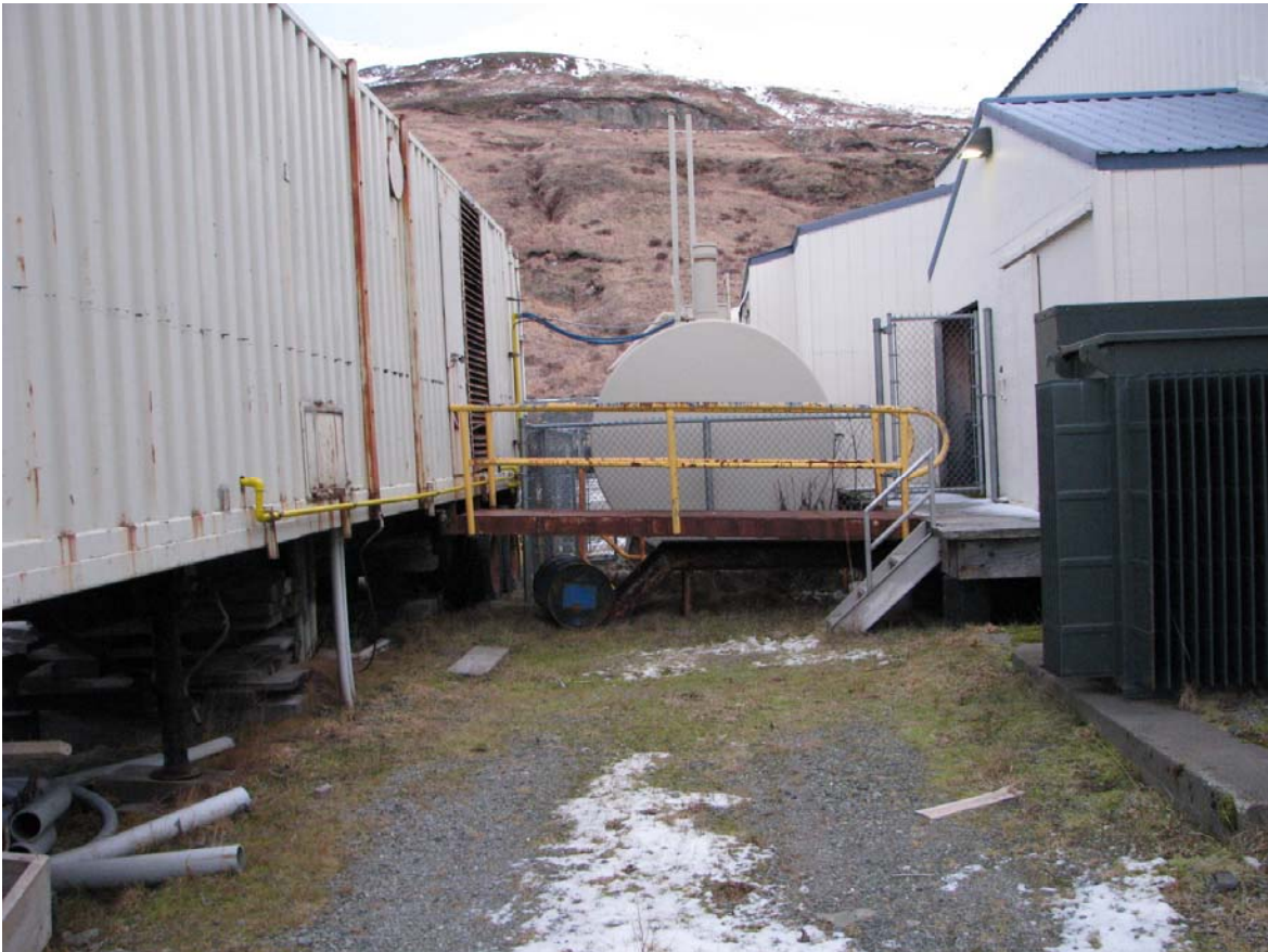
DPW Generator Van and Fuel Tank
