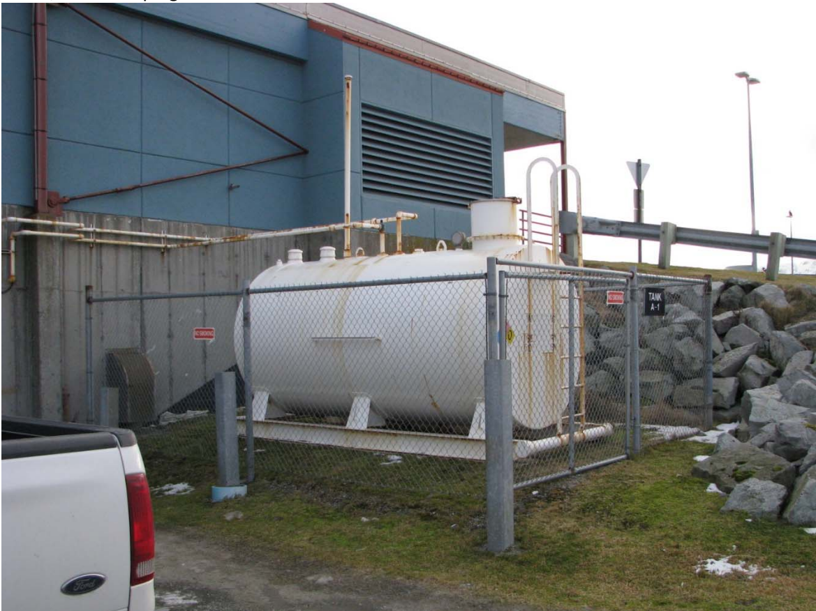
West Side, Fuel Oil Tank and Piping
