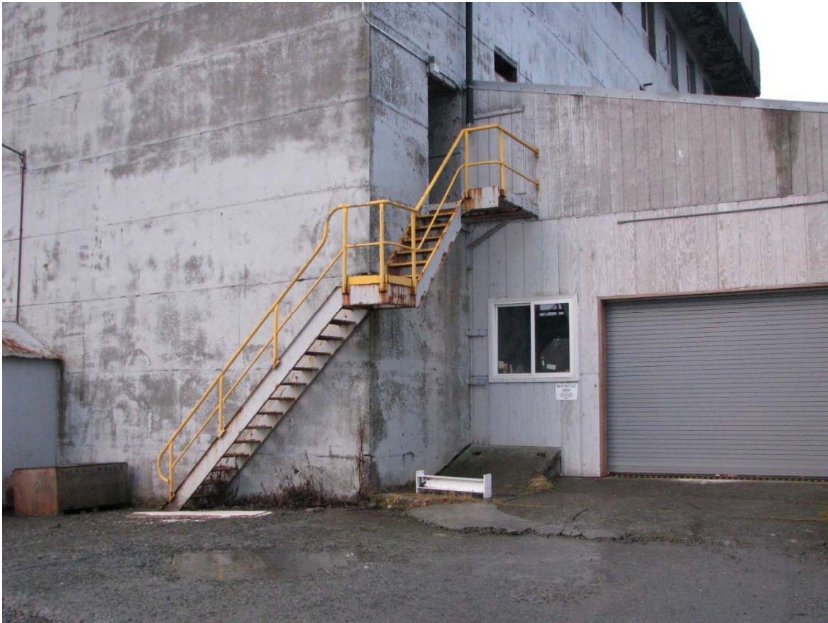
Old Powerhouse – Steel Stairs Complete (Treads, Stringers, Rails, Landings, Grating, Etc.)
