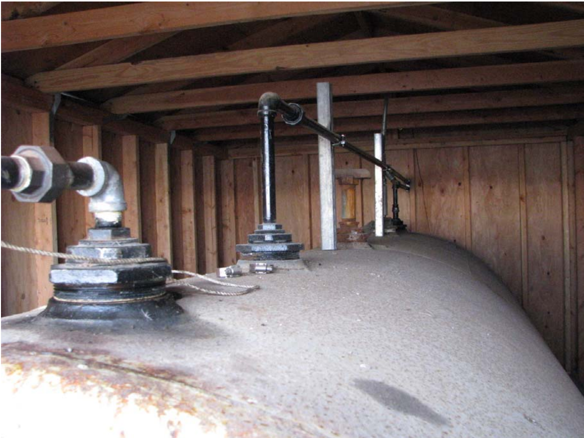
Waste Oil Tank Piping
