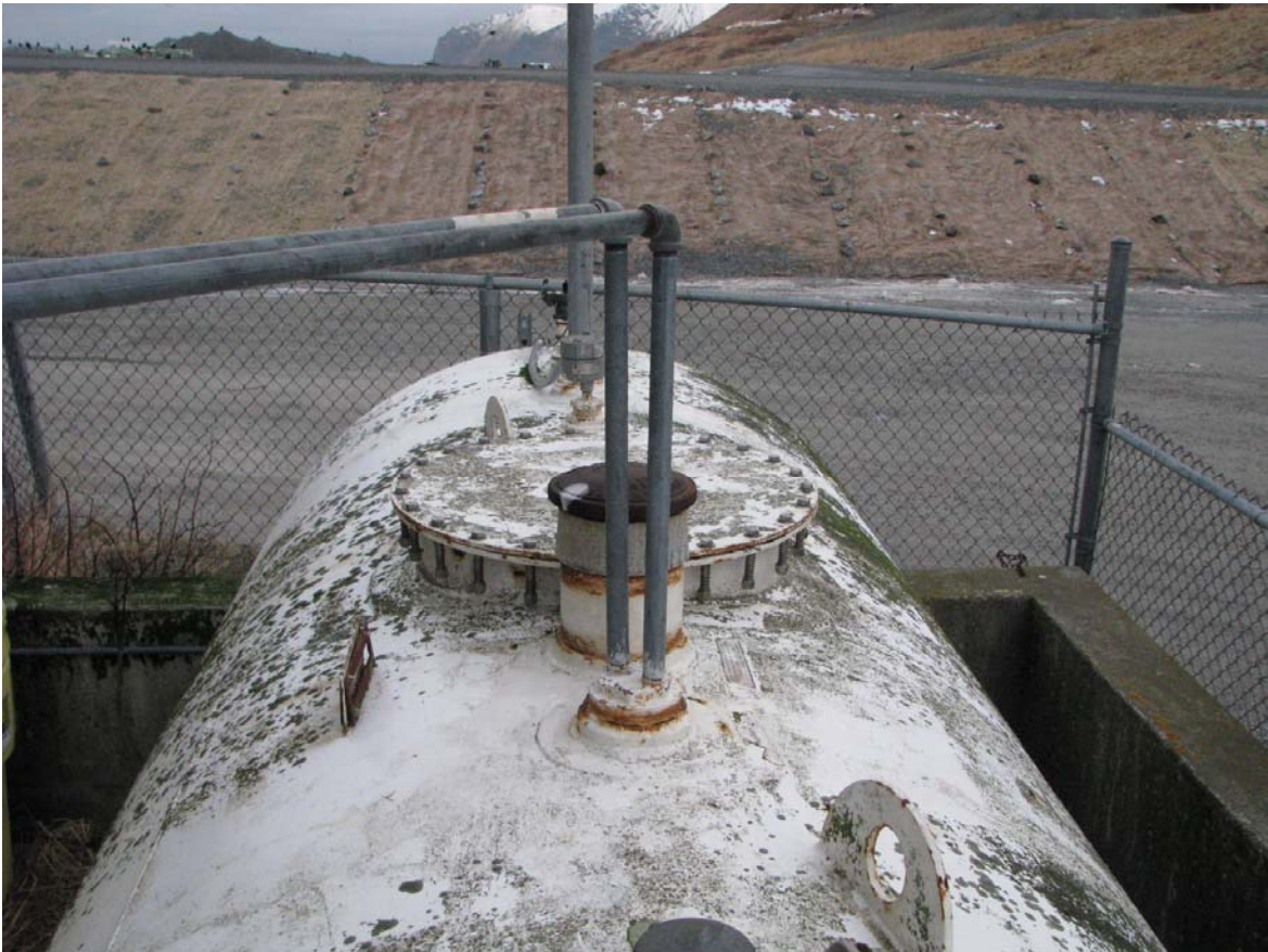
Fuel Oil Tank and Piping
