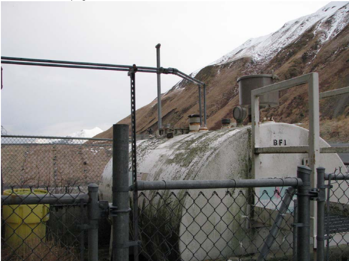
Fuel Oil Tank and Piping
