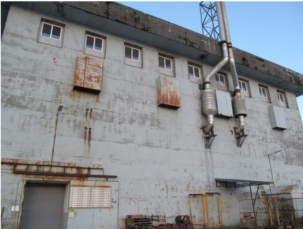
Old Powerhouse – Sheet Metal Hoods, Exhaust Stack Supports, Sliding Door
