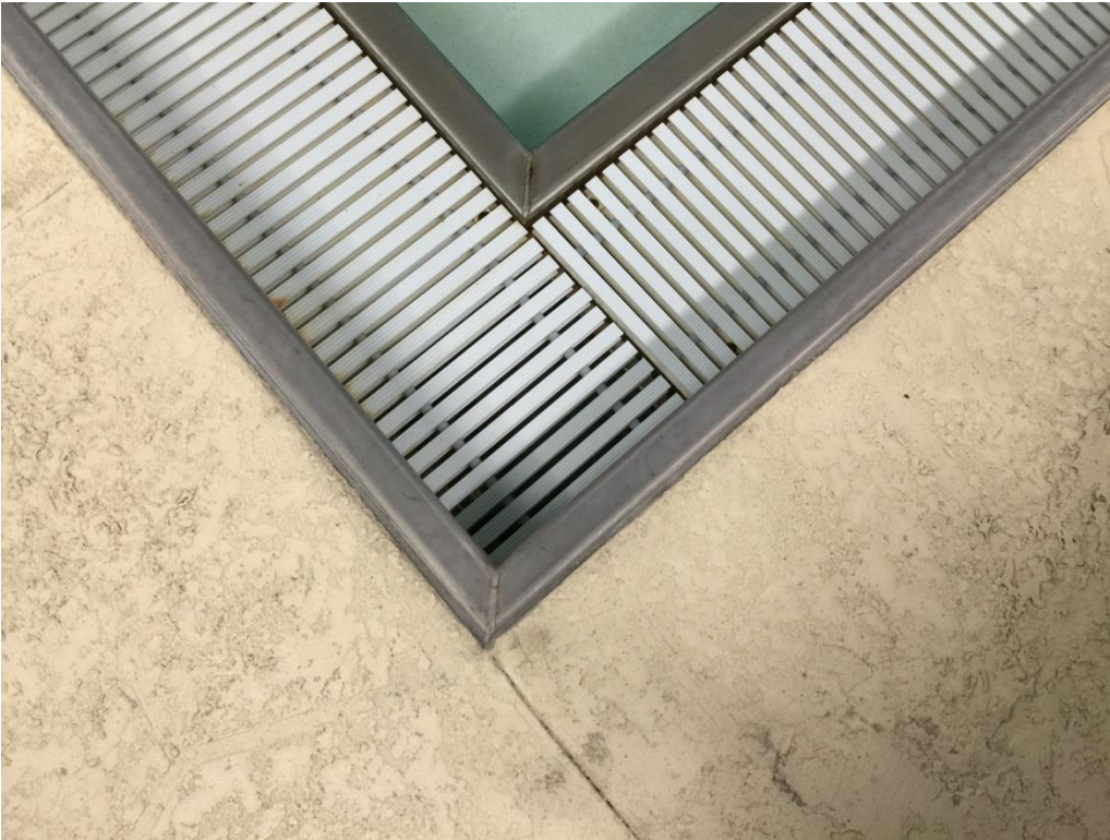
EXISTING DECKING MATERIAL INTERFACE WITH GUTTER, TYPICAL CONDITION IMAGE 5.
