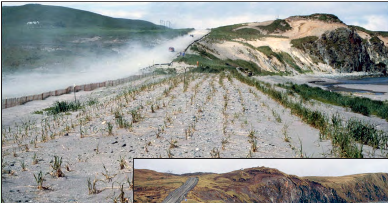
FIGURE a.24: Adak dune restoration project in 1989, 3 months after sprigging
