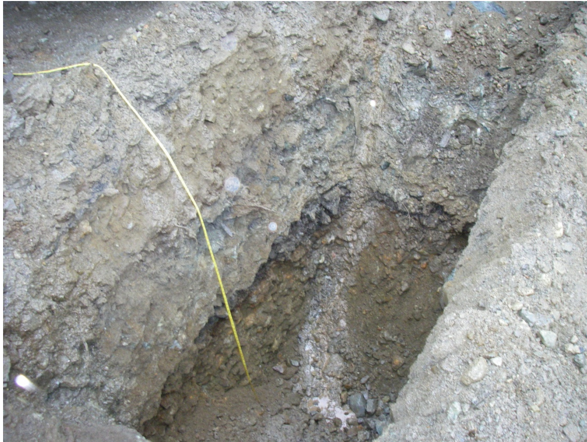
Excavated site for G10-BH02, test pit is approximately 9 feet deep. Note lighter upper layer from 0 to 5 feet depth (poorly graded gravel, shot rock fill with angular blocks to 12 inch size); and lower, rusty orange/brown layer from 5 to 9 feet depth (poorly graded gravel, "beach gravels", horizontal layering, subrounded cobbles to 6 inch size).
