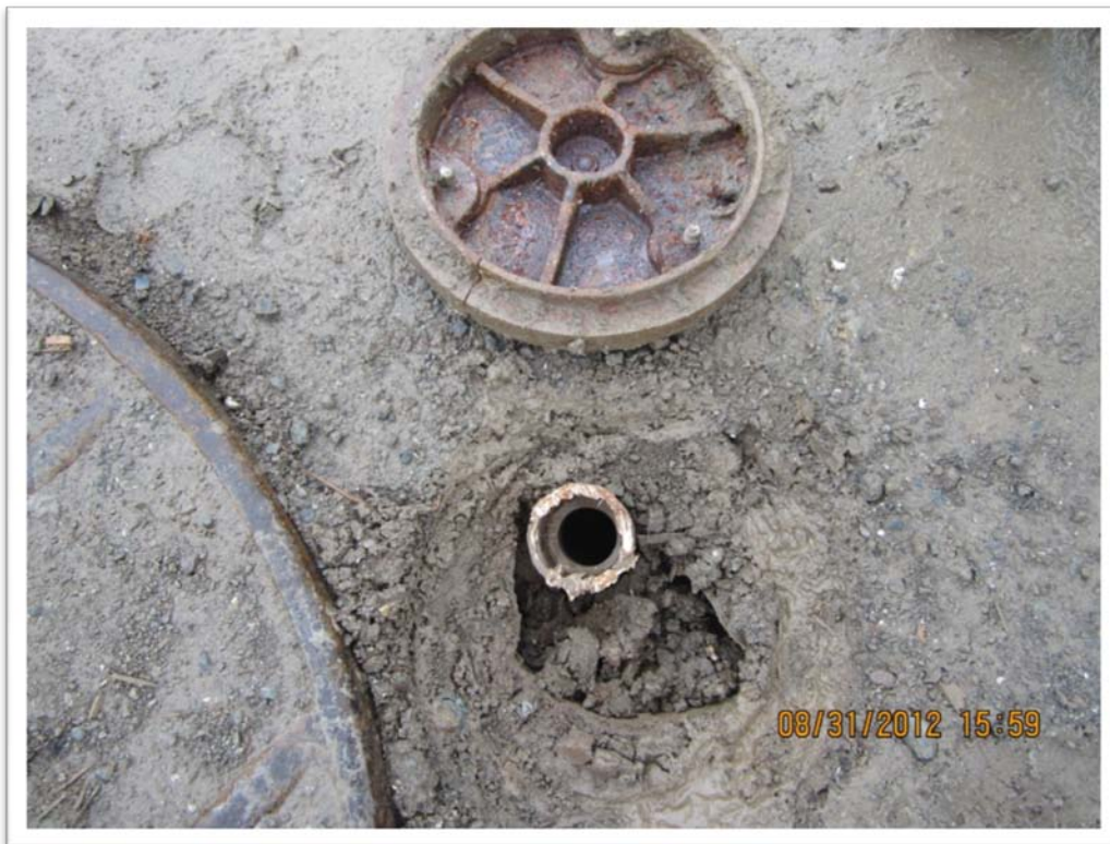
Photograph 25 – MW-18 had no cap and a destroyed monument. .
