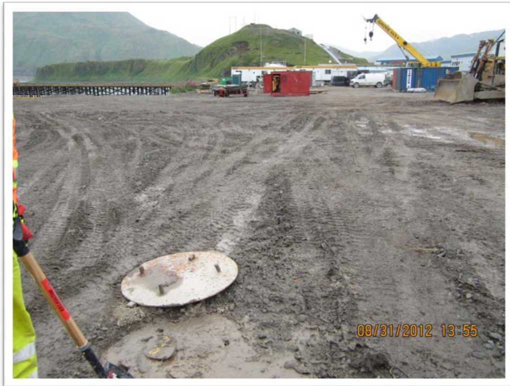
Photograph 15 – Locating well MW-11; this well was previously a stick-up, but was cut down to a flushmount during construction activities. View to the south.
