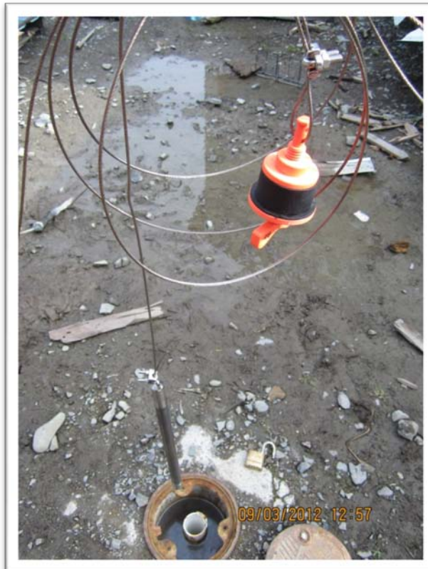
Photograph 12 – Installing transducer in MW-8R.
