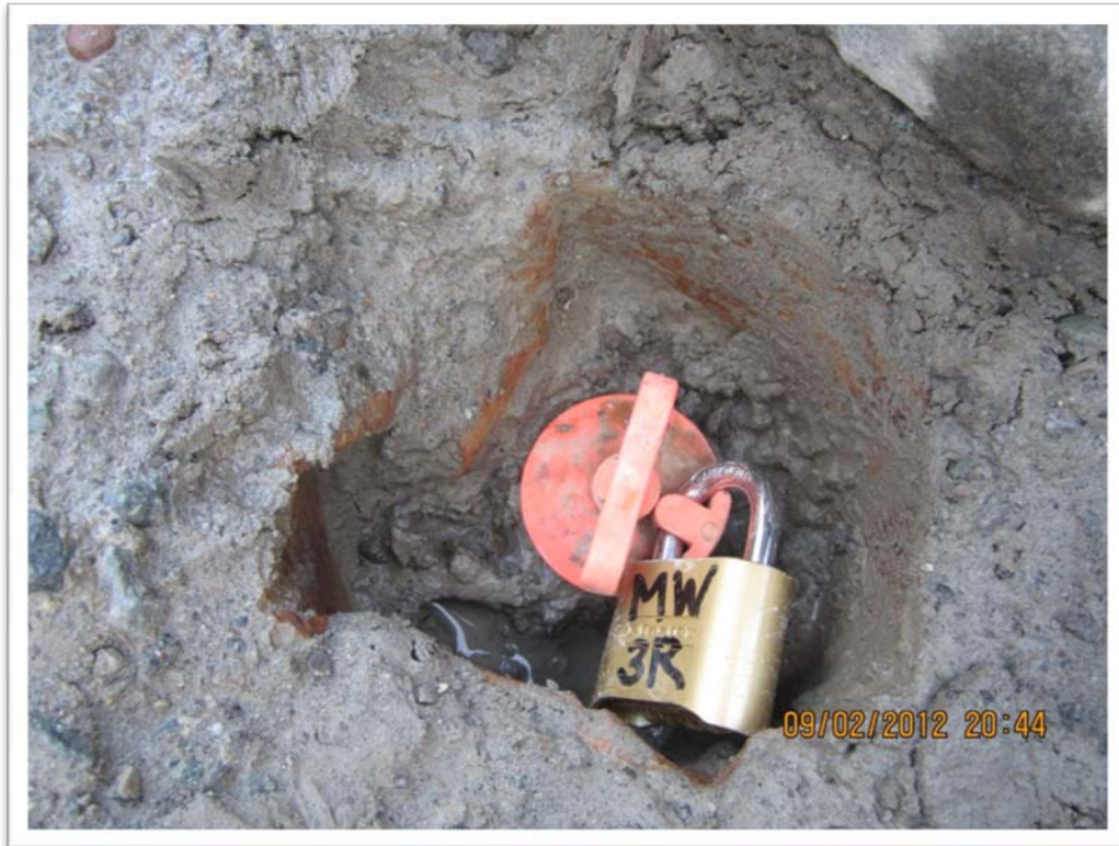
Photograph 5 – Close up shot of MW-3R, well is in poor condition with broken monument.
