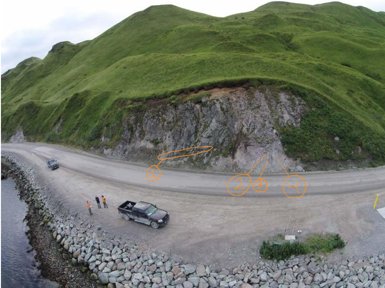
Photo 4. Wide angle view of Area 3.
