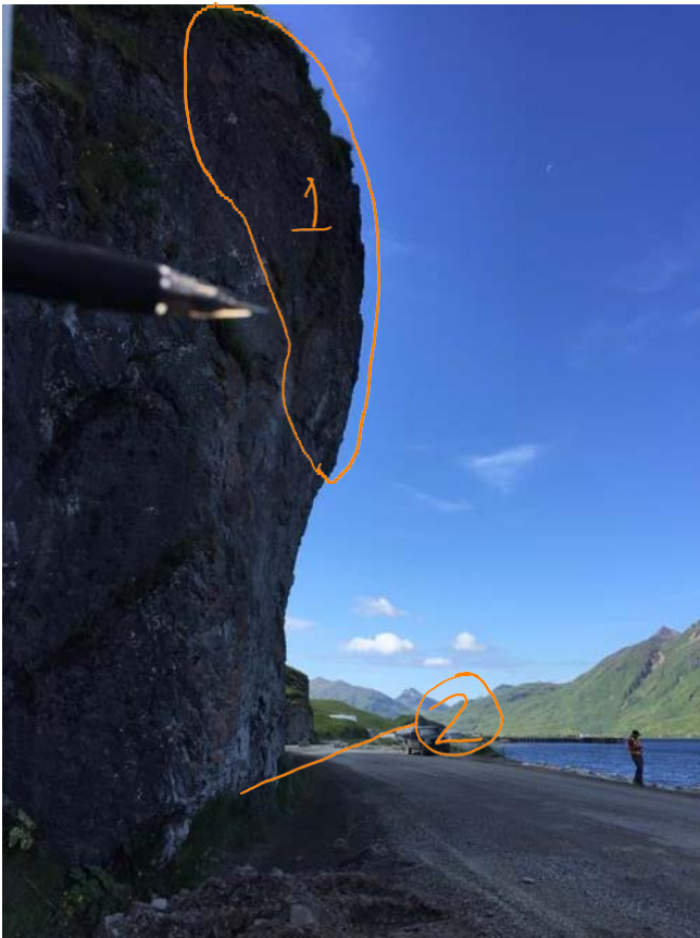
Photo 9 (Left). Looking southwest at a portion of Area 5.
