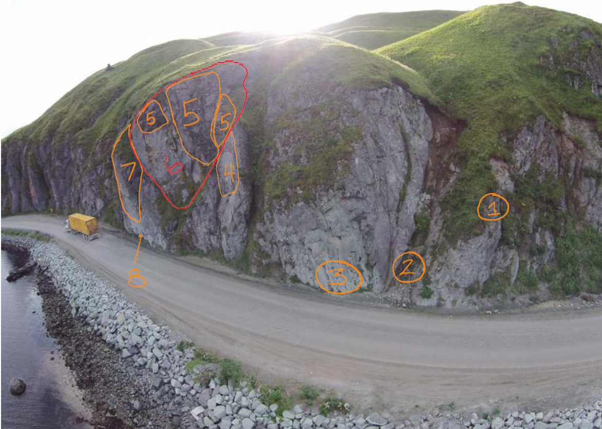
Photo 8. Wide angle view of Area 5.
