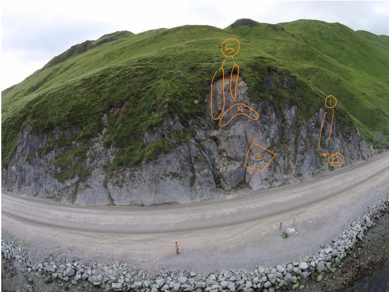
Photo 1. Wide angle view of Area 1.
