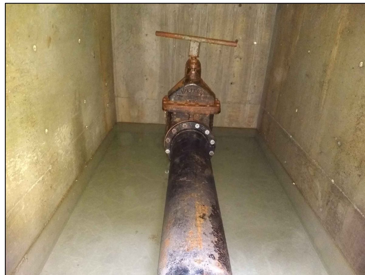
PHOTO - EXISTING VAULT AT WSI
