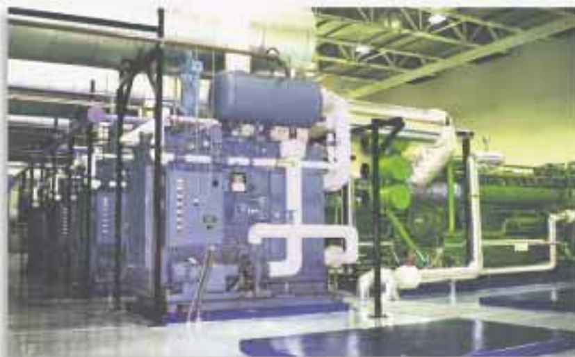
HOSPITAL , Renton, Washington (4) Model ESG1-616B19CSS Recovering Btu from (4) Jenbacher JMS-320, 900kW natural gas engines. Reducing each 2,498 SCFM from 977°F to 392°F. Delivering 1,863 pph steam @ 90 PSI operating (150 PSIG design).
