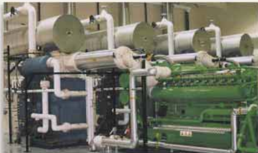
HOSPITAL , Renton, Washington (4) Model ESG1-616B19CSS Recovering Btu from (4) Jenbacher JMS-320, 900kW natural gas engines. Reducing each 2,498 SCFM from 977°F to 392°F. Delivering 1,863 pph steam @ 90 PSI operating (150 PSIG design).
