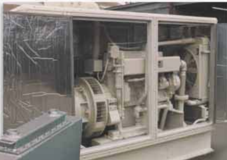
MOBILE TRAILER , Venice, California Model UTR-630218CSS. Recovering Btu from a 33kW natural gas engine. Reducing 1,282°F @ 76 SCFM to 319°F; Raising 27 GPM 50% ethylene glycol from 190°F to 198°F
