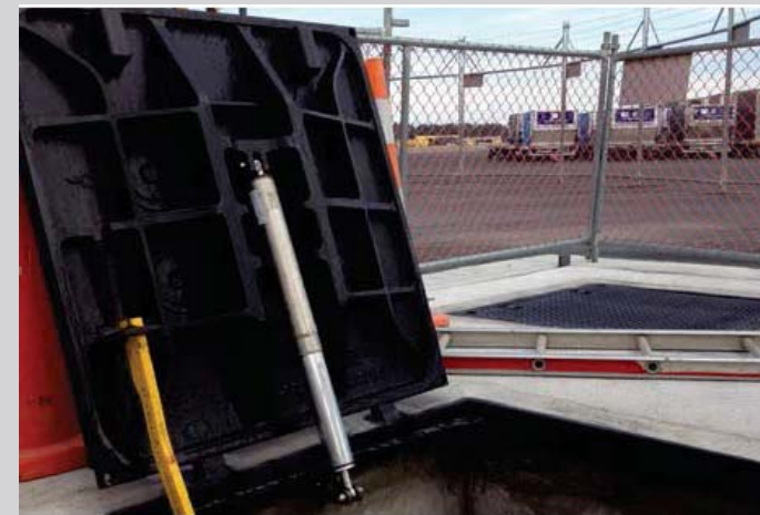
Hinged Hatch Access. Photo Courtesy of EJ Group, Inc.
