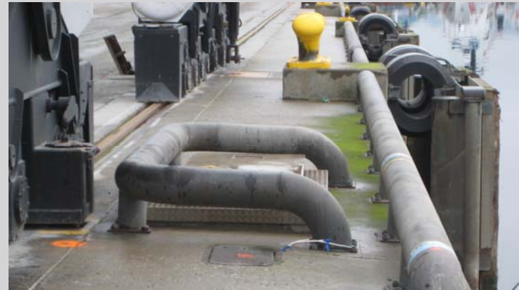
Existing Vault with Bullrails
