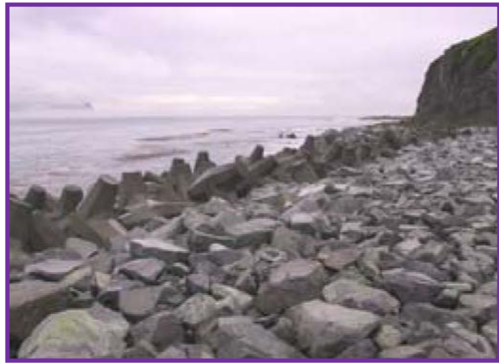
Figure 5-5 Precast Concrete Dolosse (DNR2009)
