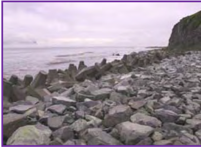
Figure 5-5 Precast Concrete Dolosse (DNR 2009)
