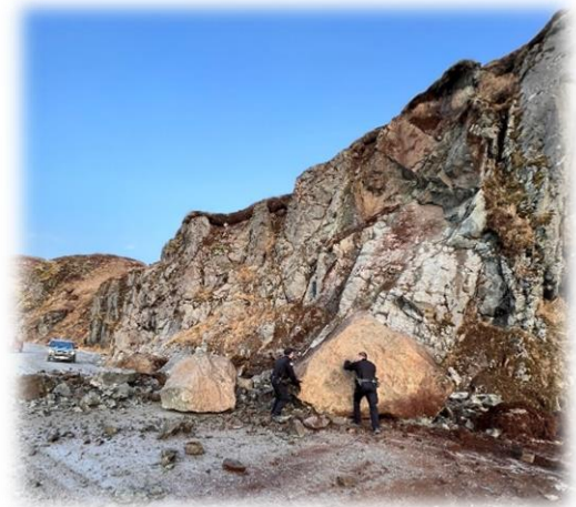
Figure 1: Three boulders totaling 36 tons fell on CBR in March 2023
