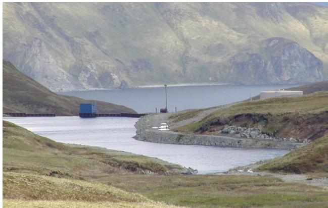
Extending the water main along Captain's Bay Road would remove a bottleneck in the water system and allow the City to use the Icy Creek Reservoir (pictured here) and Pyramid WTP to their fullest potential.
