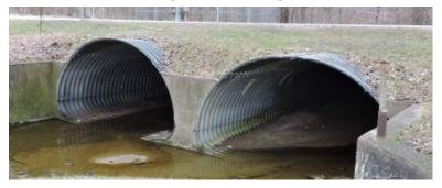
Proposed culverts improve fish habitat, can be visually inspected, and are large enough to accommodate tidal fluctuations and heavy rainfall.
