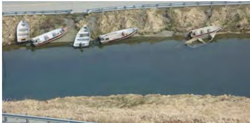
Figure 8. Middle Iliuliuk River - erosion and tramplng. May 14, 2008.
