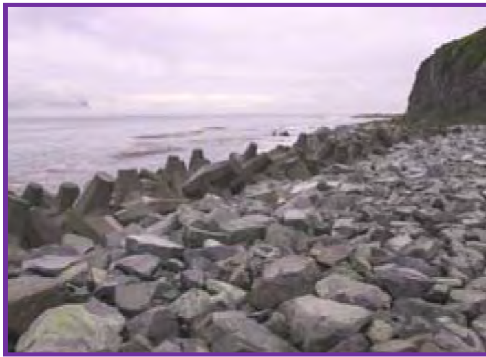
Figure 5-5 Precast Concrete Dolosse (DNR 2009)
