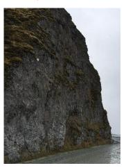
HDL will evaluate the rock slopes that may be scaled/removed for road realignment. The nature of the fracture patterns will be mapped and recommendations for reducing the potential for falling rocks to affect safety or the roadway. Catchment basins, sloping. benching, stabilization like rock bolting could be used. If needed. Landslide Technology available to provide specialty consultation on stabilizing rock
