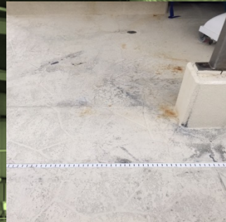
Damaged Pool Deck and Drain
